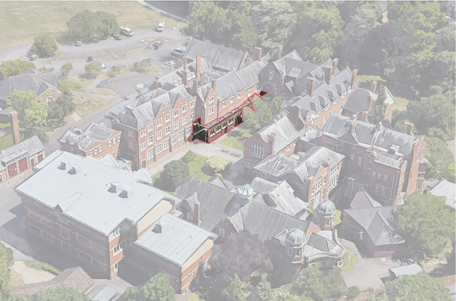
Aerial View of the Main Block
