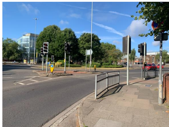
Photograph 12: Castle Street Staggered Crossing
