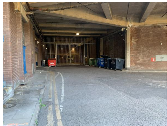
Photograph 2: Existing Basement Access
