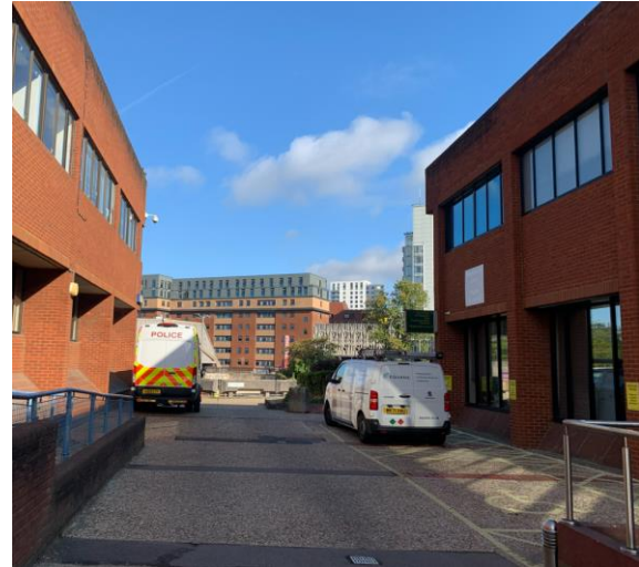
Photograph 16: Cusden Walk Existing Conditions (Facing North)
