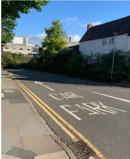
Photograph 7: Access Road Existing Conditions
