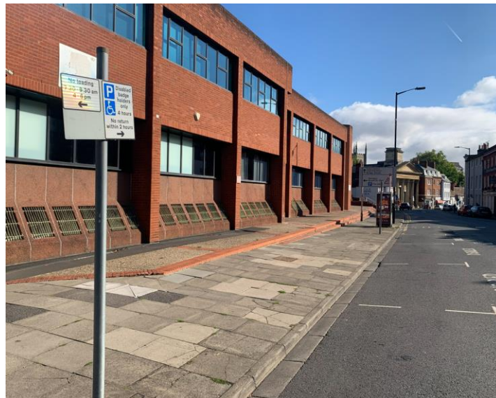
Photograph 5: Castle Street Disabled Parking Bays
