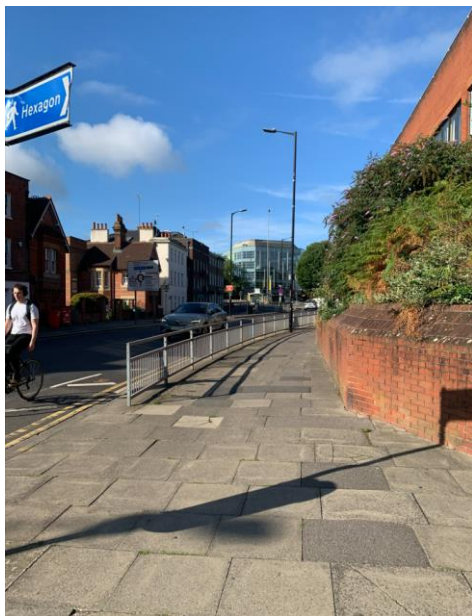
Photograph 9: Castle Street Northern Footway Conditions
