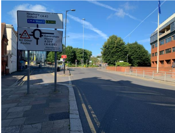
Photograph 3: Castle Street Existing Conditions (Facing West)
