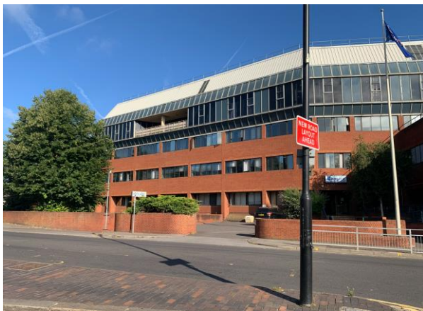
Photograph 1: Existing Site Frontage on Castle Street
