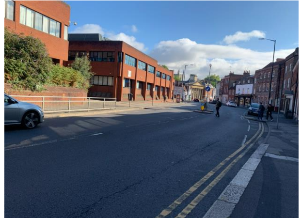
Photograph 4: Castle Street Existing Conditions (Facing East)
