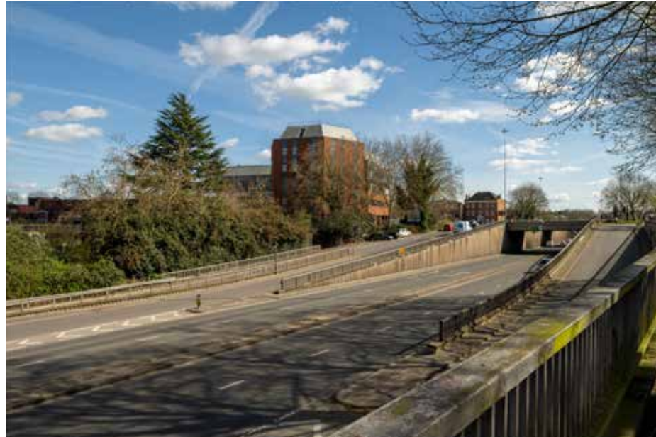
Figure 7.8 View 1: Howard Street/Baker Street – existing (EB7)
