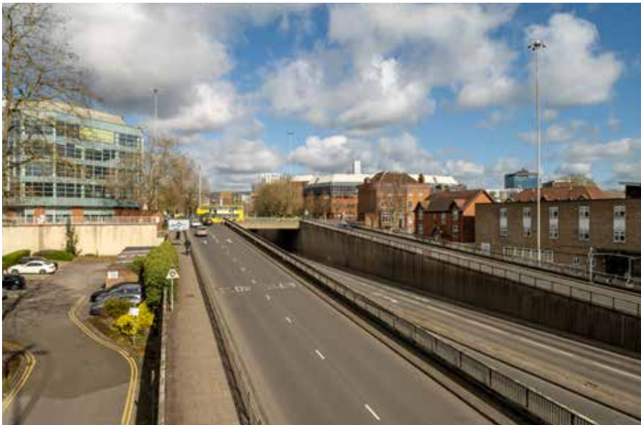
Figure 7.12 View 12: Footbridge over A329 – existing (EB7)
