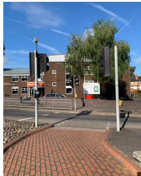
Photograph 14: 4-Arm Roundabout Signalised Crossing
