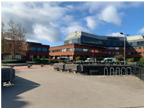
Photograph 17: San Francisco Libre Walk Existing Conditions (Facing South)
