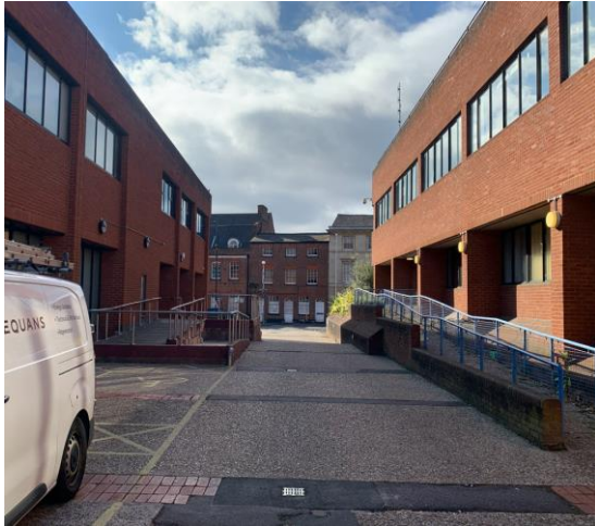
Photograph 15: Cusden Walk Existing Conditions (Facing South)
