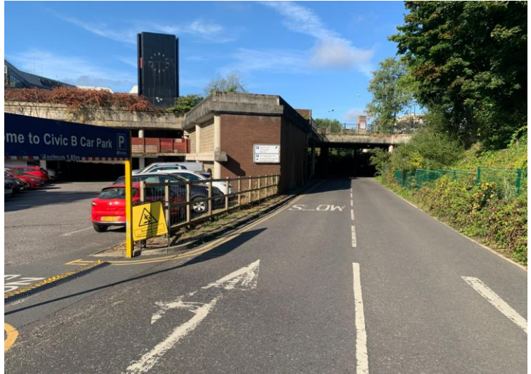
Photograph 8: Access Road Existing Conditions
