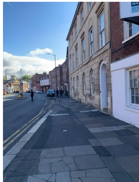
Photograph 10: Castle Street Southern Footway Conditions
