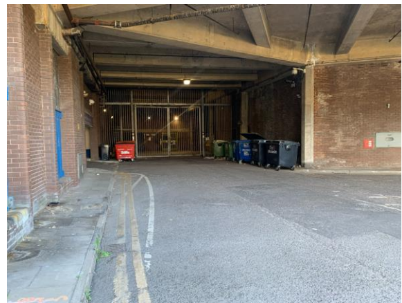
Photograph 2: Existing Basement Access
