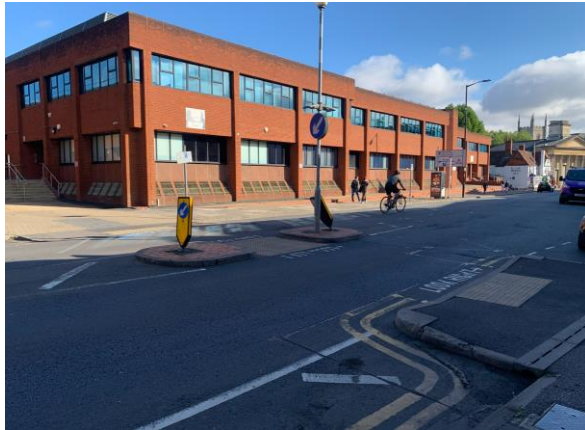
Photograph 11: Castle Street Pedestrian Refuge Island Crossing
