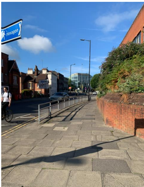
Photograph 9: Castle Street Northern Footway Conditions
