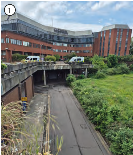
Rear. Existing service road access to basement
