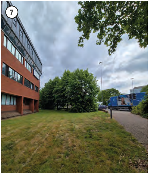
Existing trees along the site frontage interfacing with roundabout
