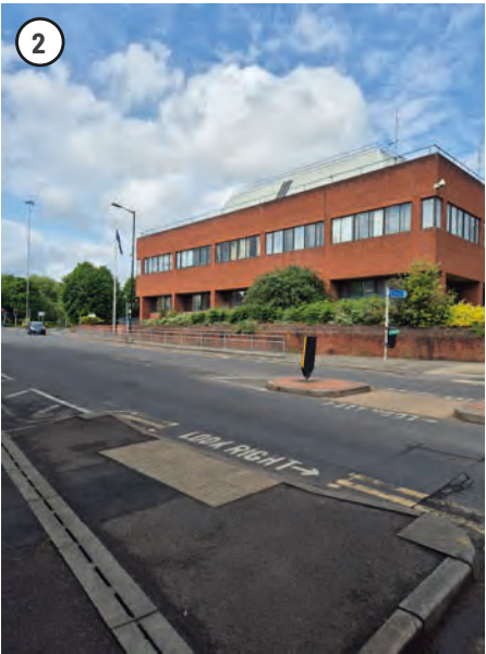
View from pedestrian crossing on Castle Street
