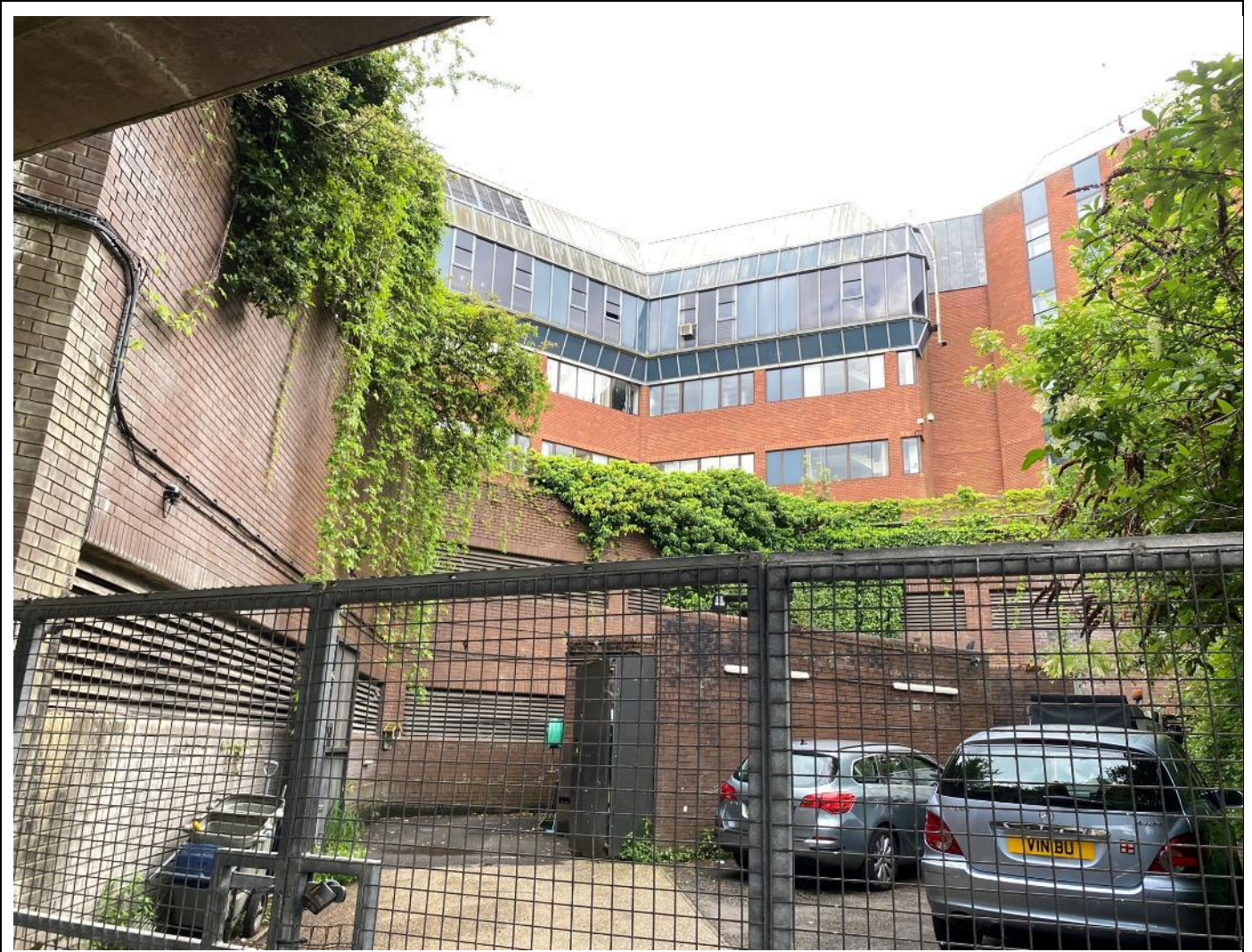
Image 5: South facing view of Reading Police Station from the lower basement level.
