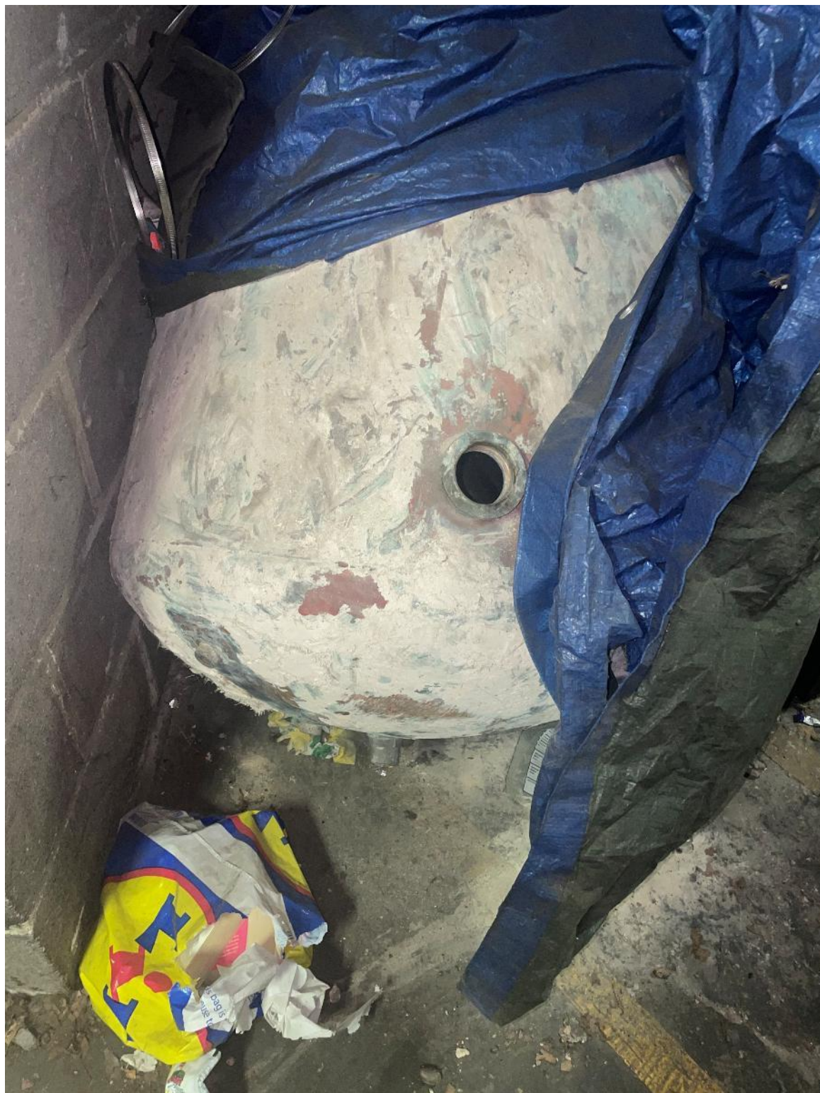
Image 8: Unidentified tank located in basement level
