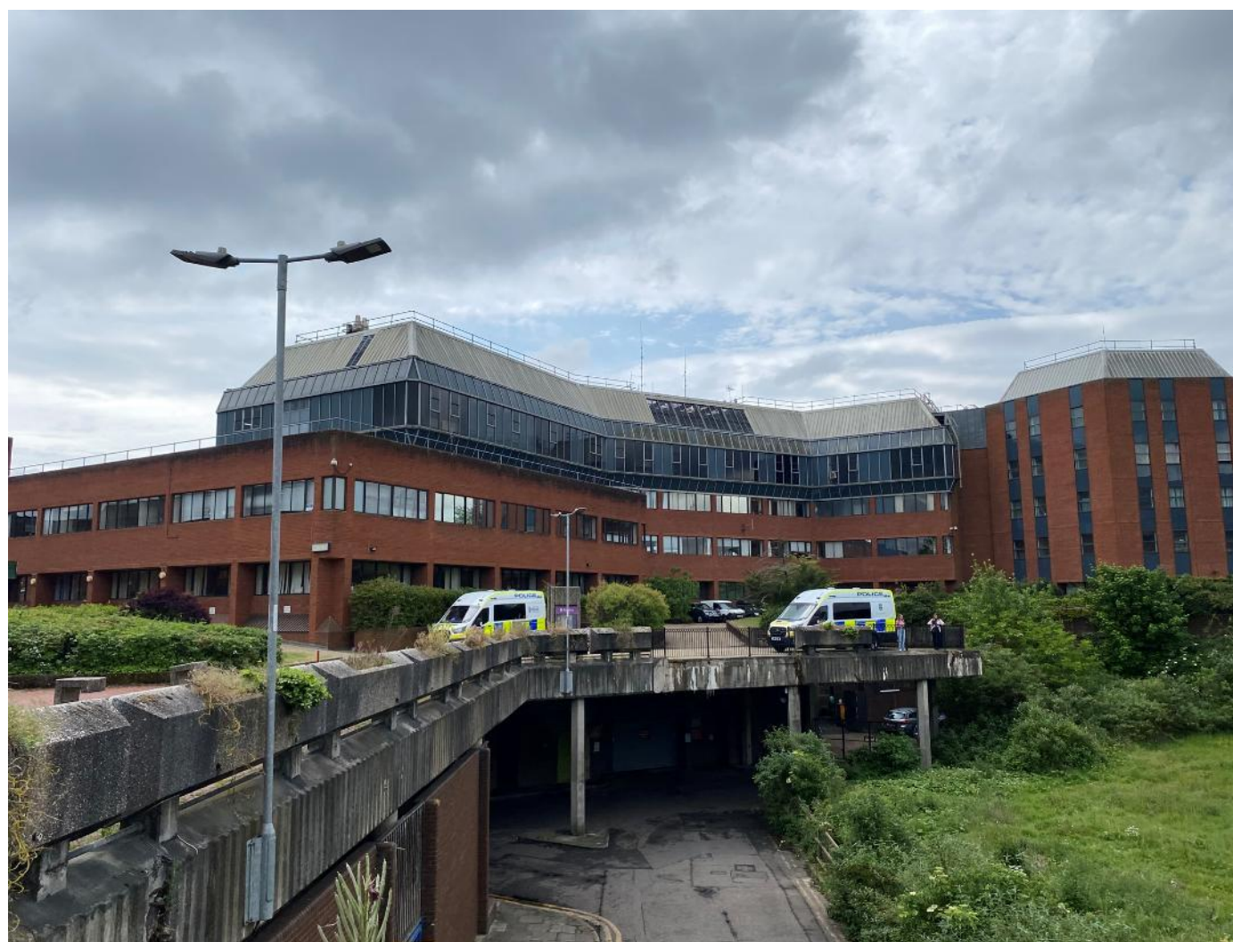
Image 1: Reading Police Station south facing view.
