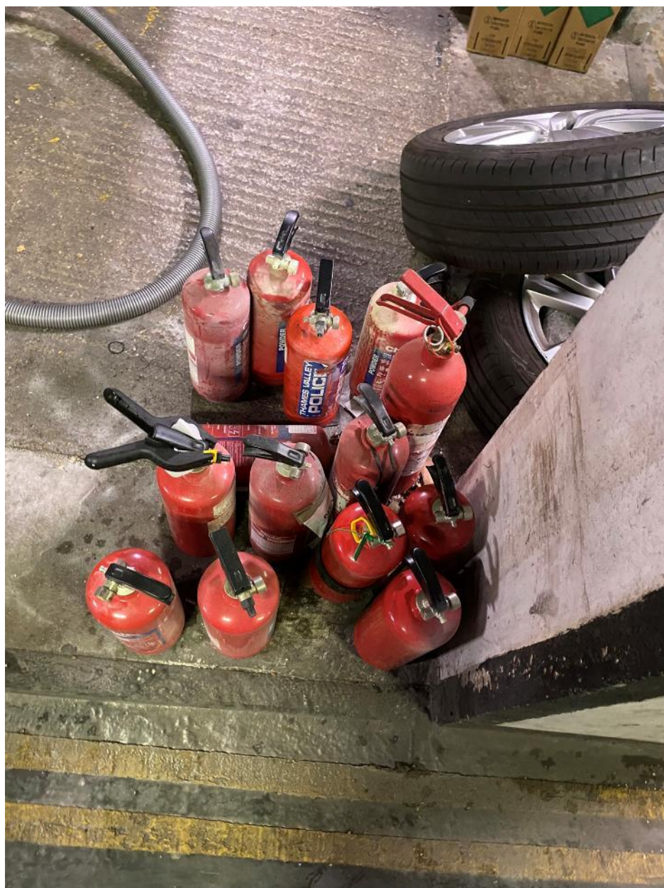
Image 4: Fire Extinguishers being kept directly on the ground.
