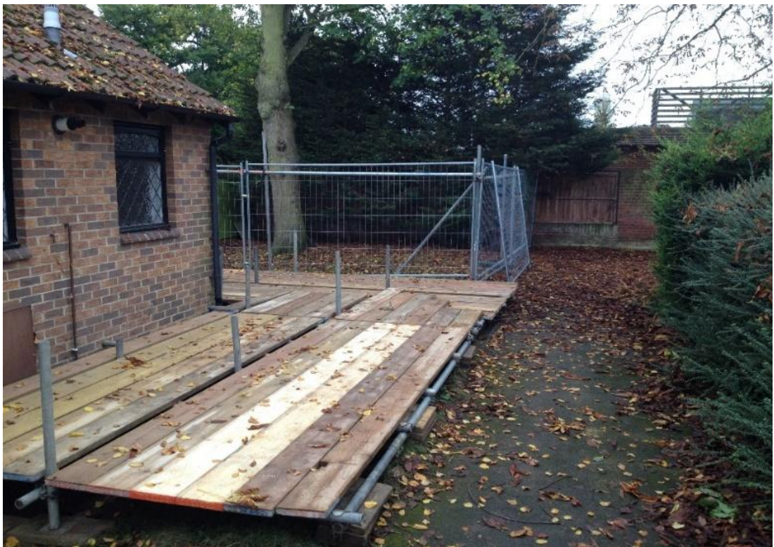
Figure 9 – Specification for scaffold ground protection
