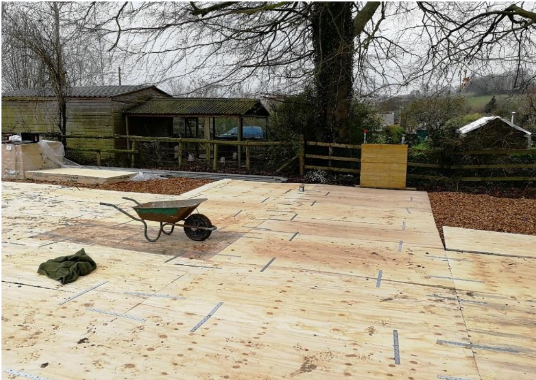
Figure 8 – Plywood sheeting used as ground protection
