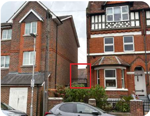
Partial View between Pheonix Place/5 Waylen Street
