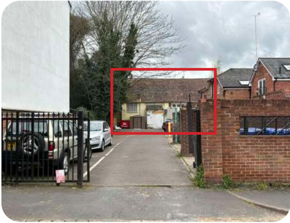
Russell Hall Site Entry Via Zinzan Street
