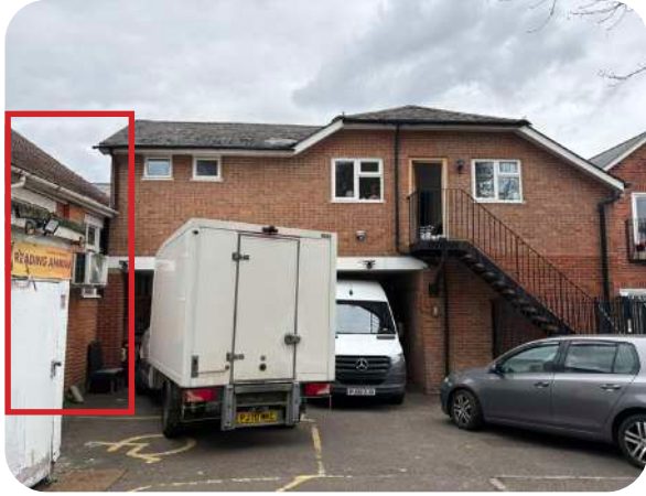
Rear Outrigger/ Undercroft Parking to Russell House
