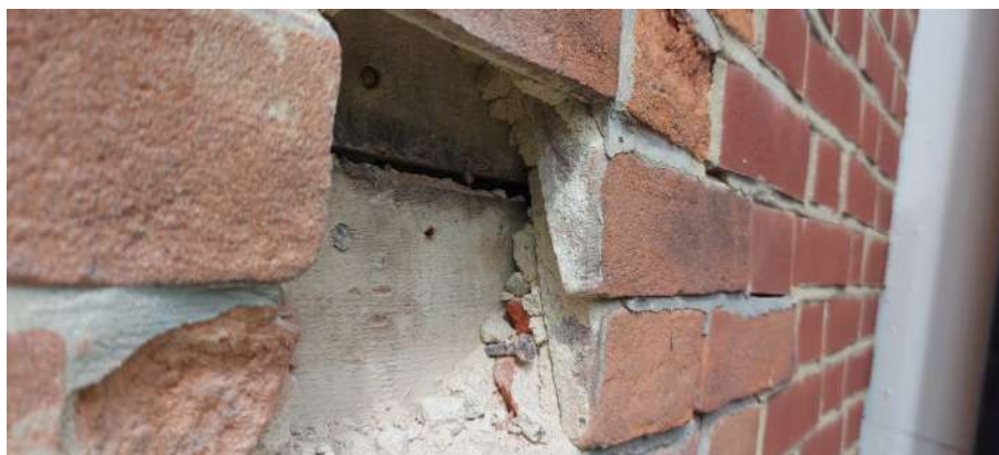
Figure 4. Detail at position in figure 3
