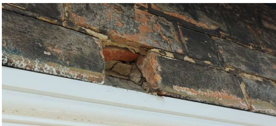
Figure 5. Top of wall – over window
