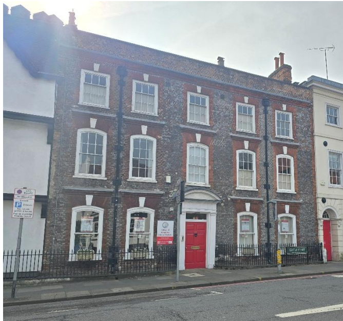
Fig 16 – Frontage of 19 Castle Street – Photograph taken by Applicant/Agent
