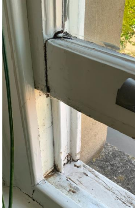
Rot to the lower sash LHS bottom rail and stile joint
