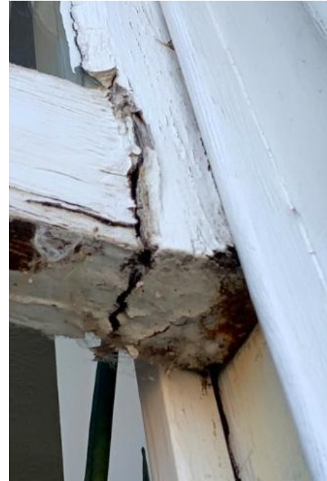
Rot to the lower sash LHS bottom rail and stile joint
