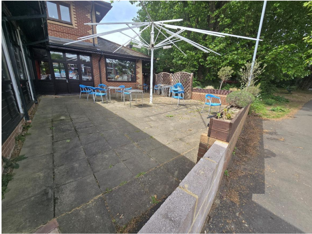
Photo 4 – Northern patio area. Shallow footings for 600x600 pad foundations will be excavated 200mm deep into the subbase of the patio. Pad positions will be lined with a non-porous membrane before concrete is poured.
