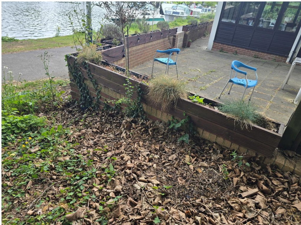
Photo 3 – Existing low-level brick retaining wall along the northern patio area.
