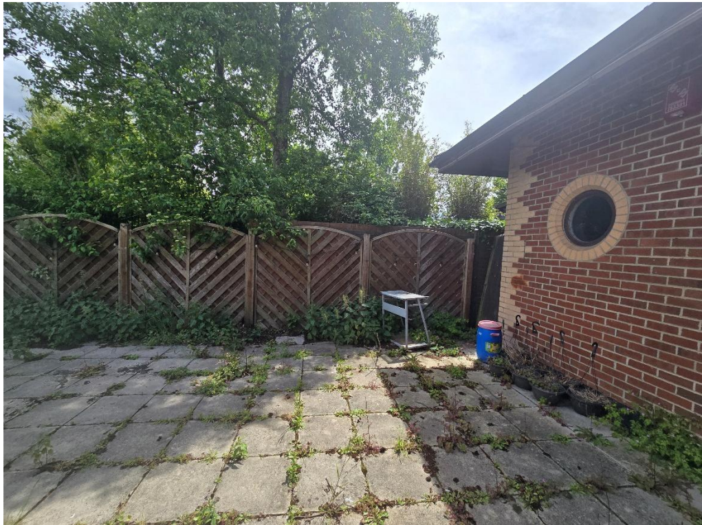
Photo 2 – Southern patio area. A substantial brick retaining wall and changes in ground levels along the southern boundary will prevent the roots of T005 & T006 (Alder) extending into the property curtilage
