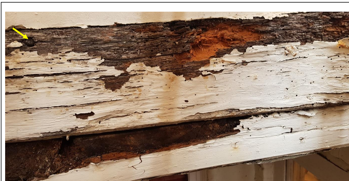
Photograph 1 Lintel (top) and associated timbers beneath it . Note wood boring insect emergence holes through white coating and coating flaking away from timbers. Surface of lintel 'picked away' revealing wood boring insect tunnels. Note peg in hole (arrowed)
