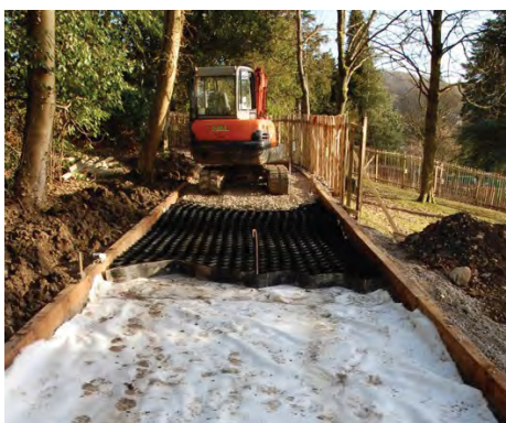
Fallbarrow Park, Windermere: CellWeb TRP® Installation
