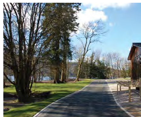
Fallbarrow Park, Windermere: Completed CellWeb TRP® Installation
