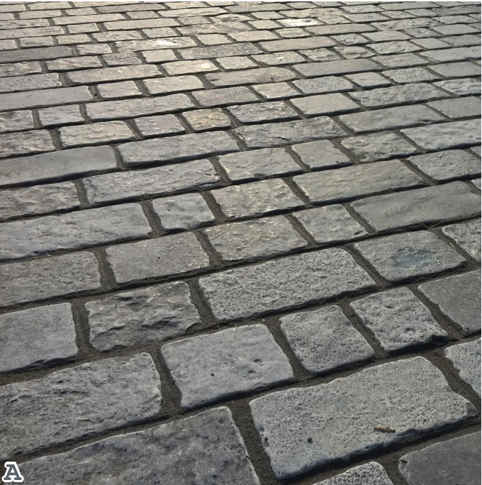
A Shared Surface - Rustic cobblestone-style stone paving in mixed dark greys. Varied stone sizes and aged finish to create a traditional reclaimed appearance
