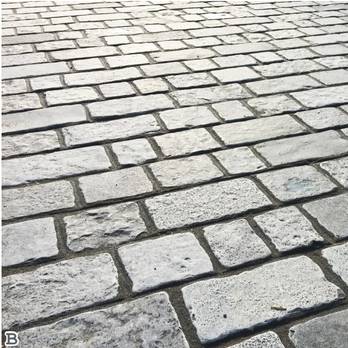
B Parking Spaces - Rustic cobblestone-style stone paving in mixed light greys. Varied stone sizes and aged finish to create a traditional reclaimed appearance
