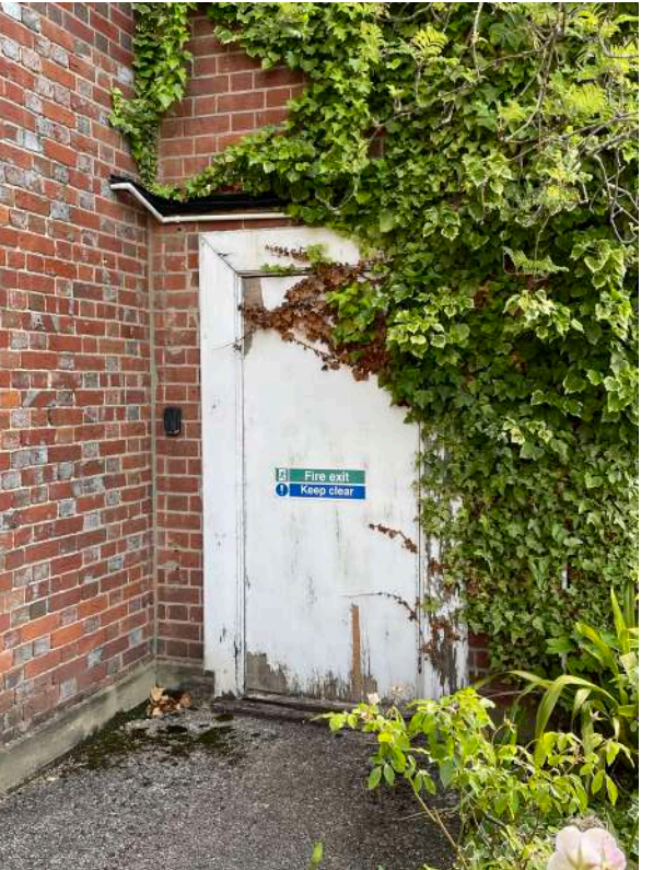
T8 - Eastern rear exit, proposed as garden access door to unit 8.
