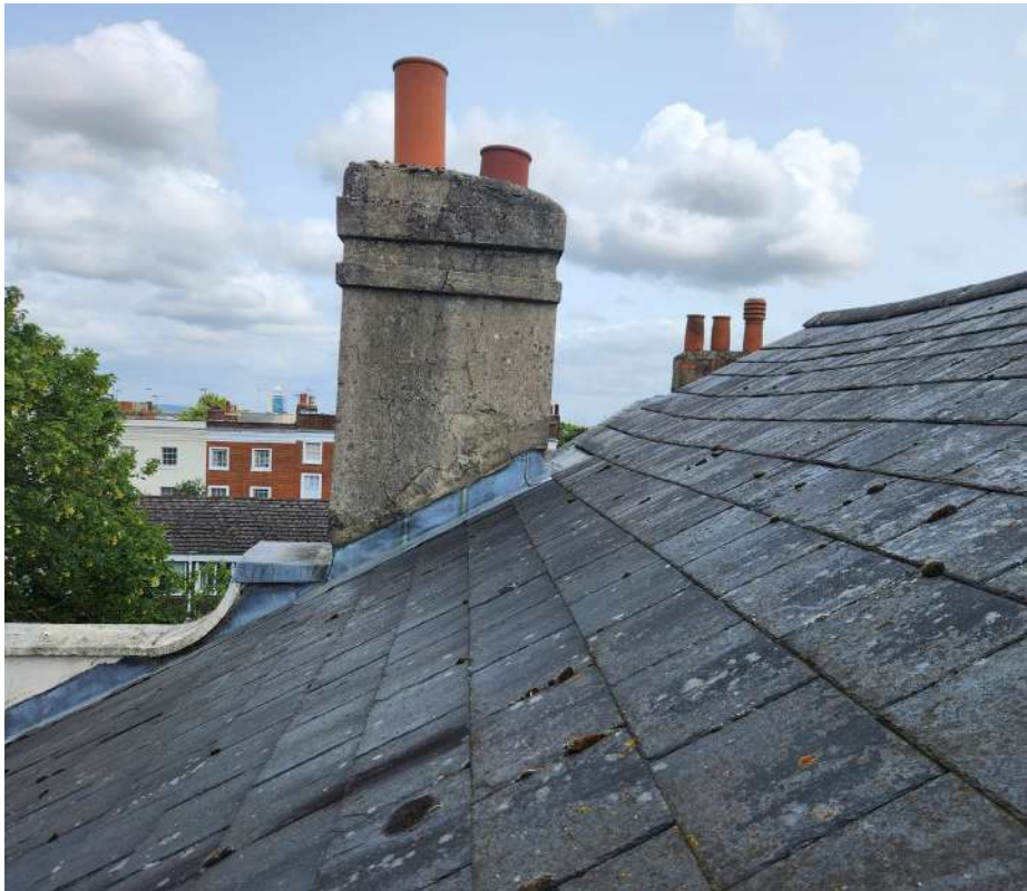
A3 - view east out of roof hatch in western storeroom (17)
