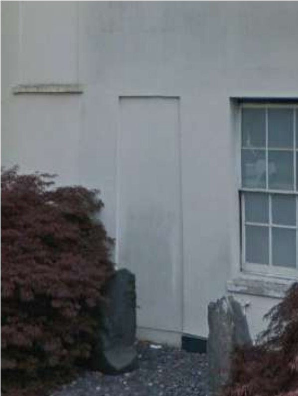
T2 - Historically blocked up doorway to be reintroduced as entrance of unit 6.
