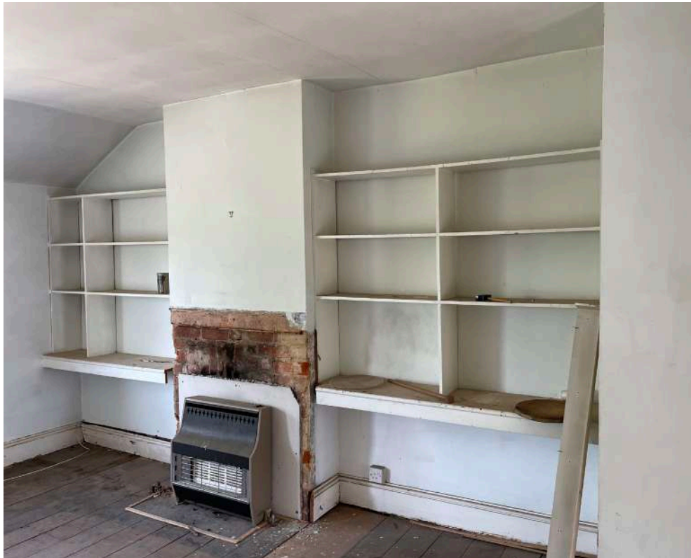
Q3.4 - modern electric heater to be removed in central room (35)
