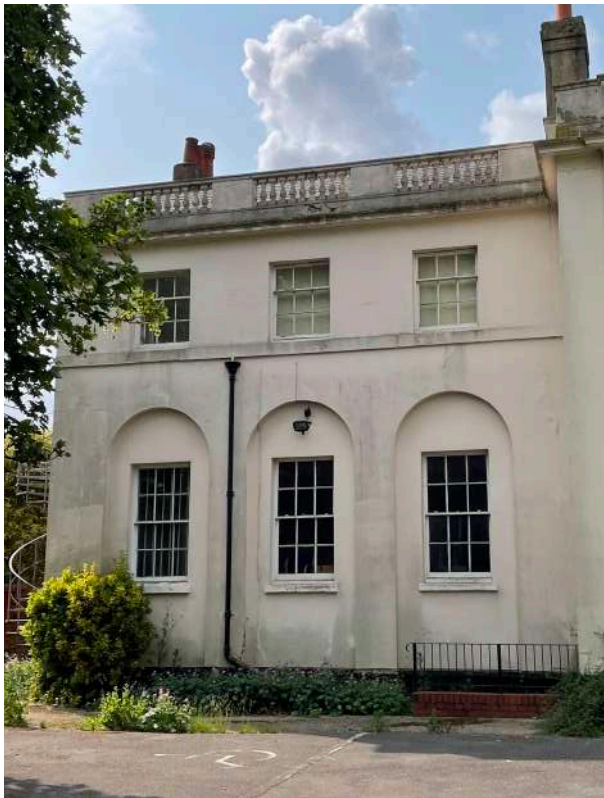
K4 - North facade with white stucco render with arches
