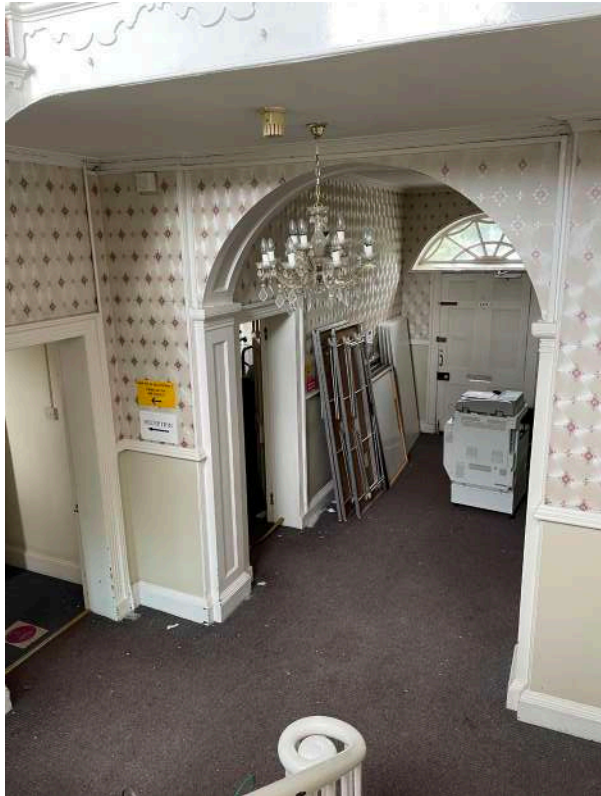
R4 - Arch shown with pilasters and panelling (1A)
