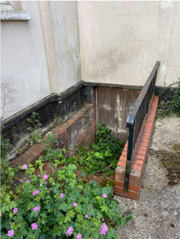
U4 - External basement stair
