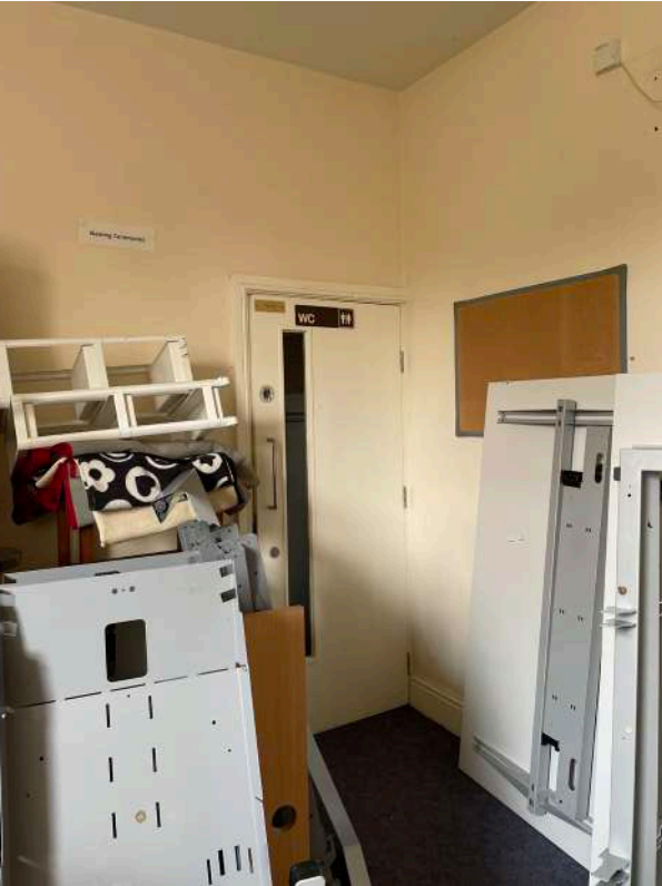
H6 - lack of cornice and modern door in waiting room (6) to be blocked up.
