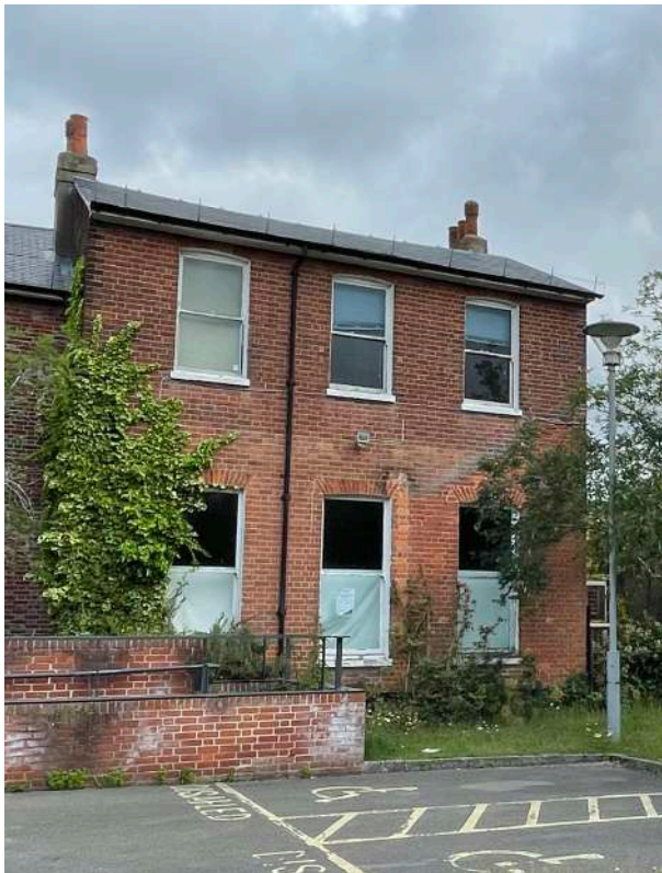
K5 - Red bricks South facade
