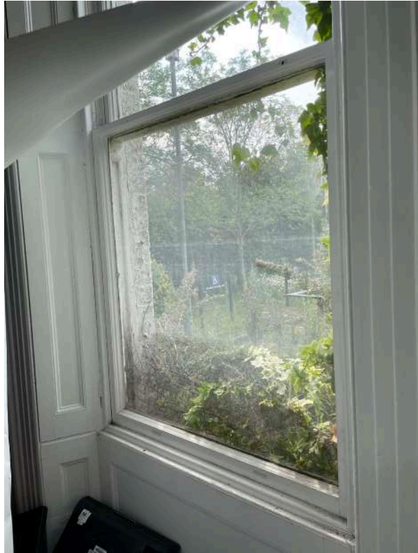
L1.8 - modern sash window, shutters and surround in large ceremony room (41)
