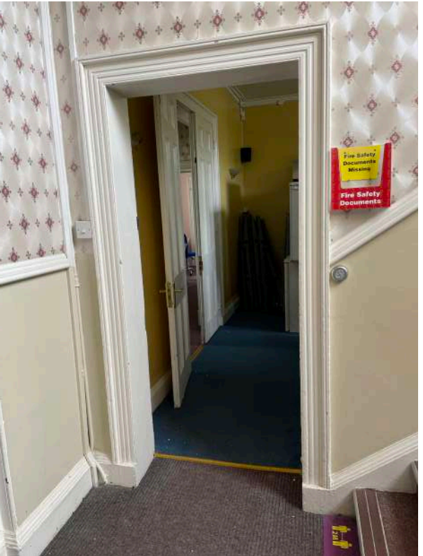
R5 - Door and architrave to the small ceremony room (1A)
