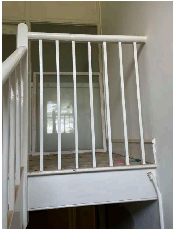
01.5 - handrail on second floor on the landing (30)
