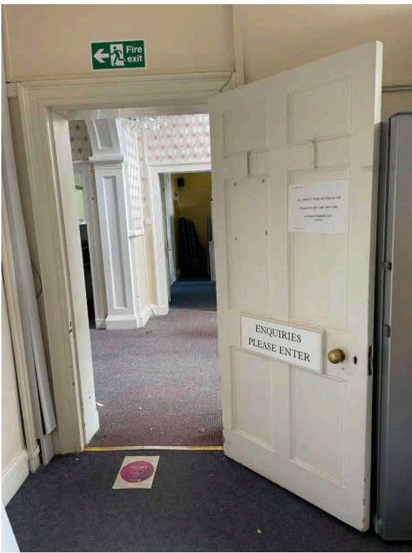
H4 - door between waiting room (6) and entrance hall (1A)
