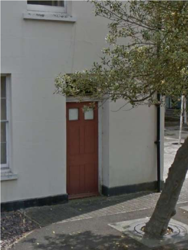
T3 - secondary front entrance, proposed as entrance to unit 7.
