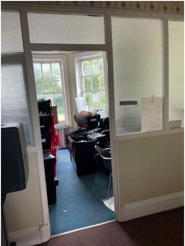
J4 - Modern glass partition between Corridor (2) and Deputy Office (3)
