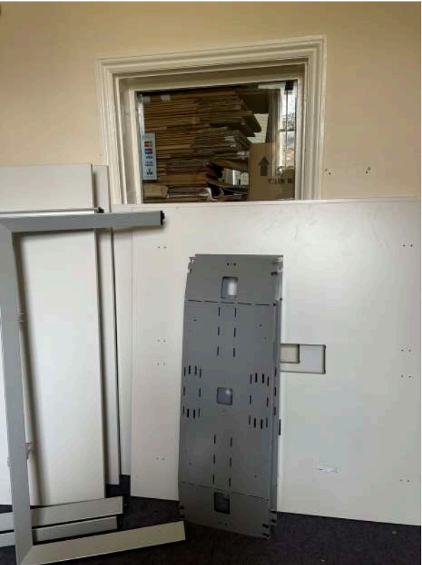
H7 - Modern window between waiting room (6) and administration office (5)
