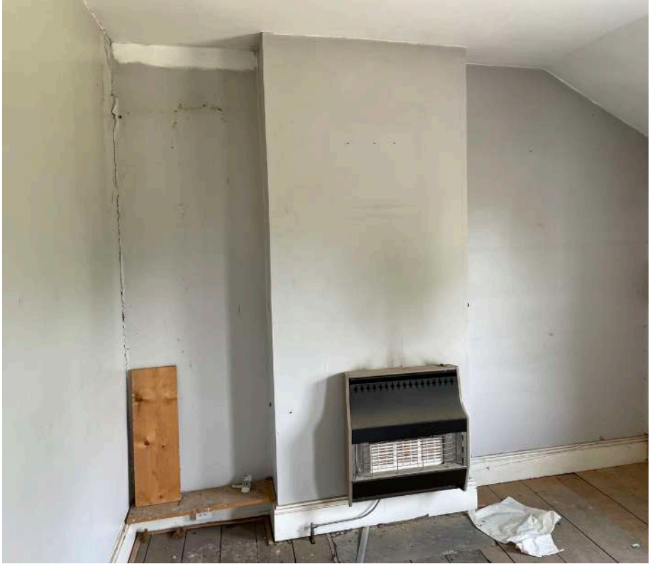
03.6 - modern electric heater to be removed from east room (31)
