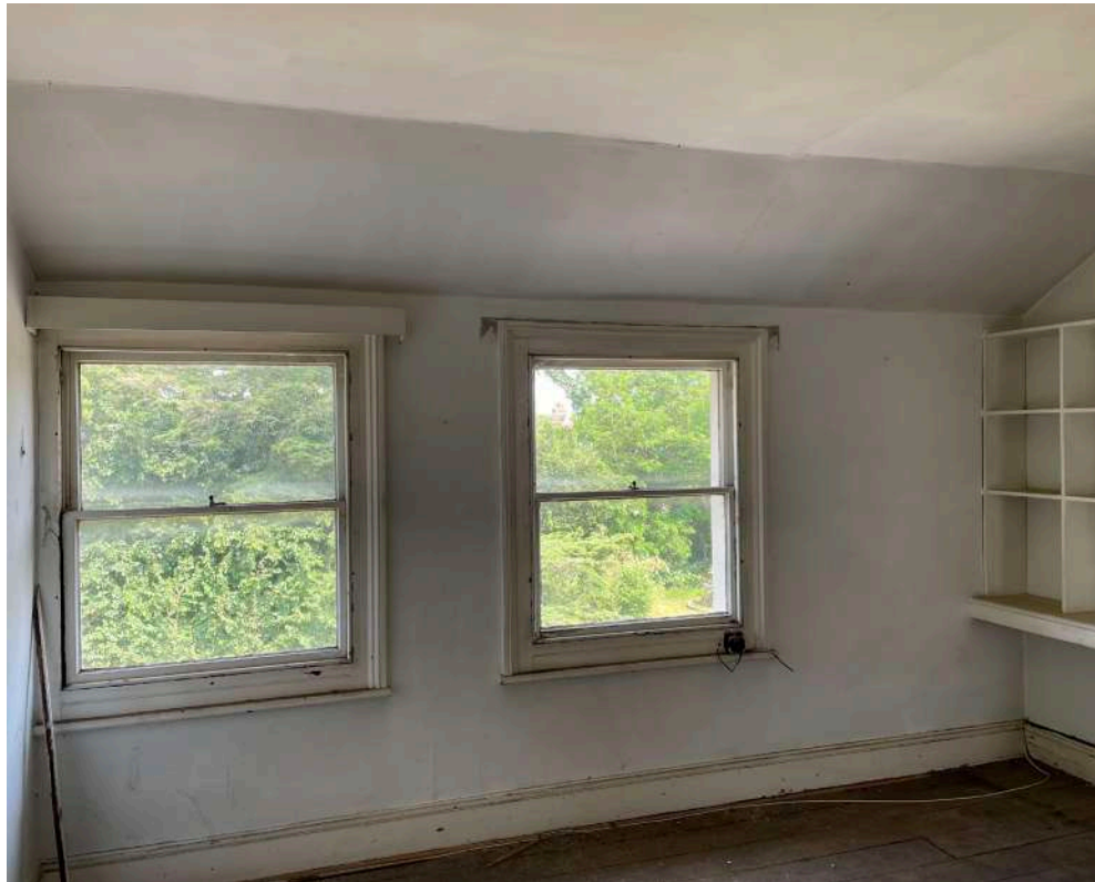
Q3.5 - sash windows and modern window architrave in central room (35)
