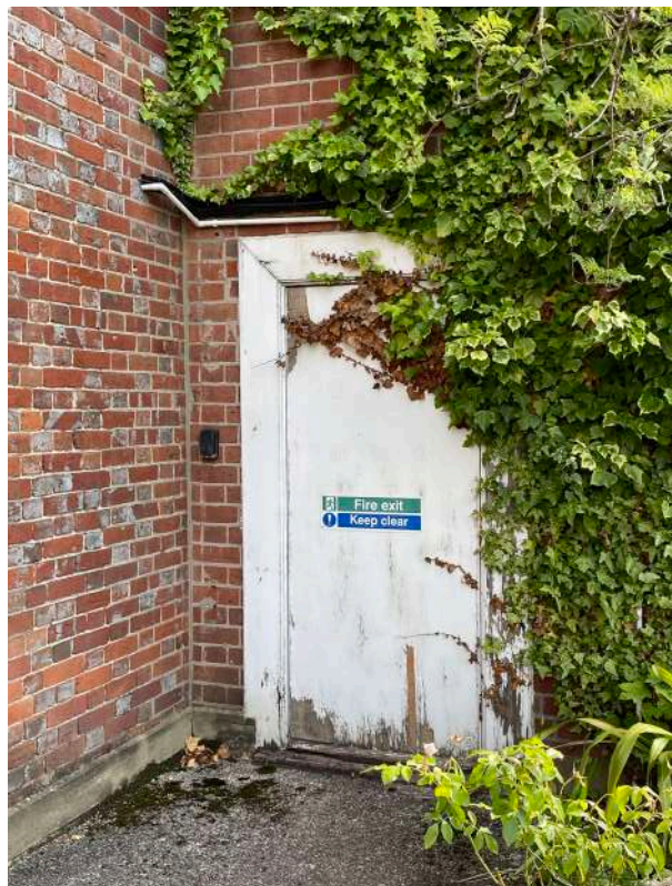
K6 - South/West facade with fire escape door
