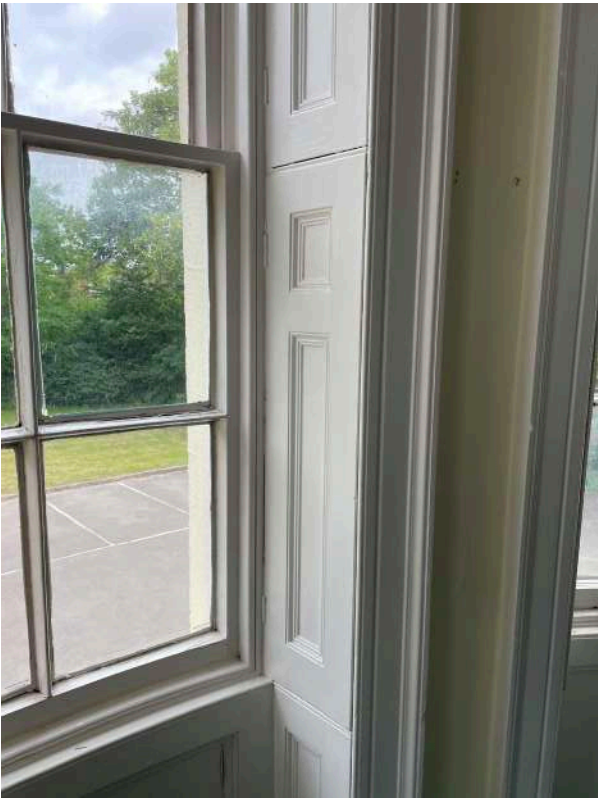
F4 - shutters in the bay window of Office A (10)
