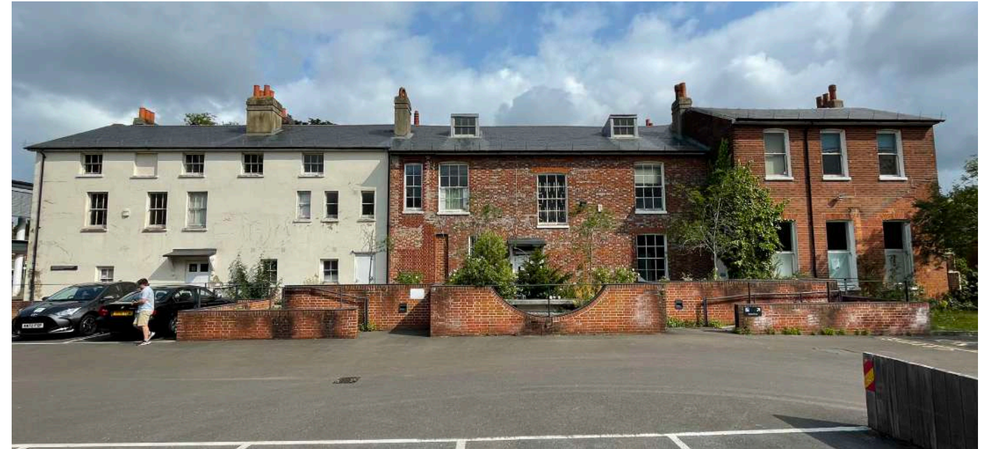
Rear Facade, Footpath Access and Drive
