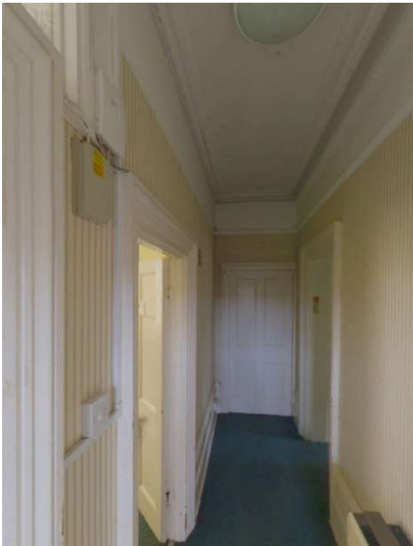
L2.10 - mismatched cornice suggests modern partition between corridor (42) and offices A (44) & B
