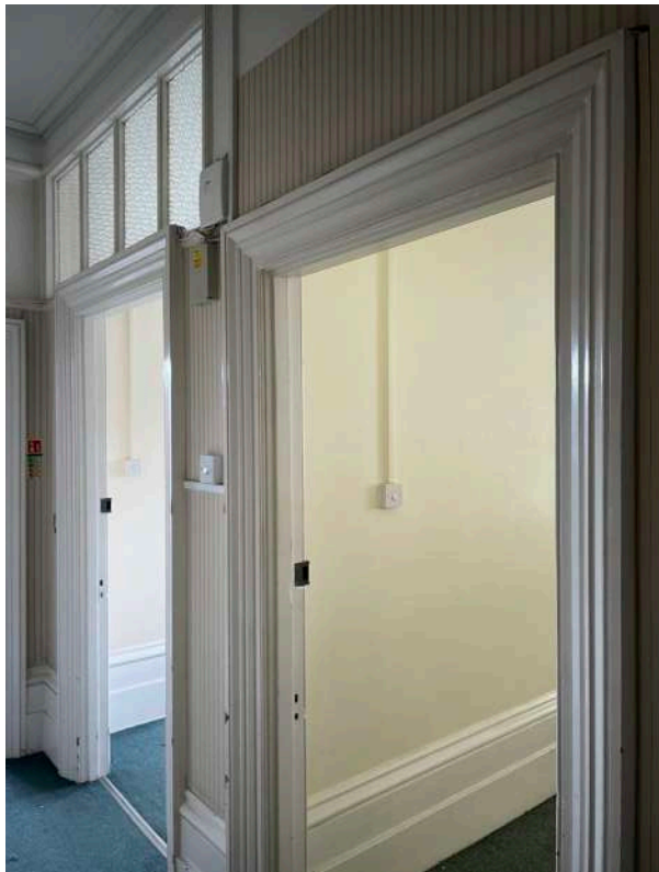
L2.11 - decorative architrave, high skirtings and services on suspected modern partition (42)
