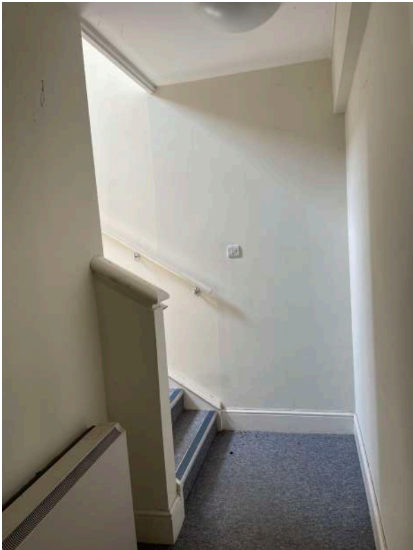
Q1.6 - modern ground to first floor stair in corridor (19)
