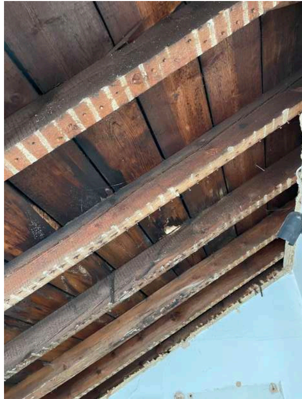
Q3.2 - exposed roof structure
