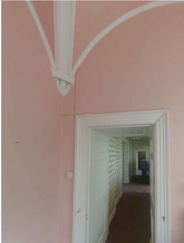
L1.7 elaborately dressed doorway between the anteroom (38) and corridor (2)
