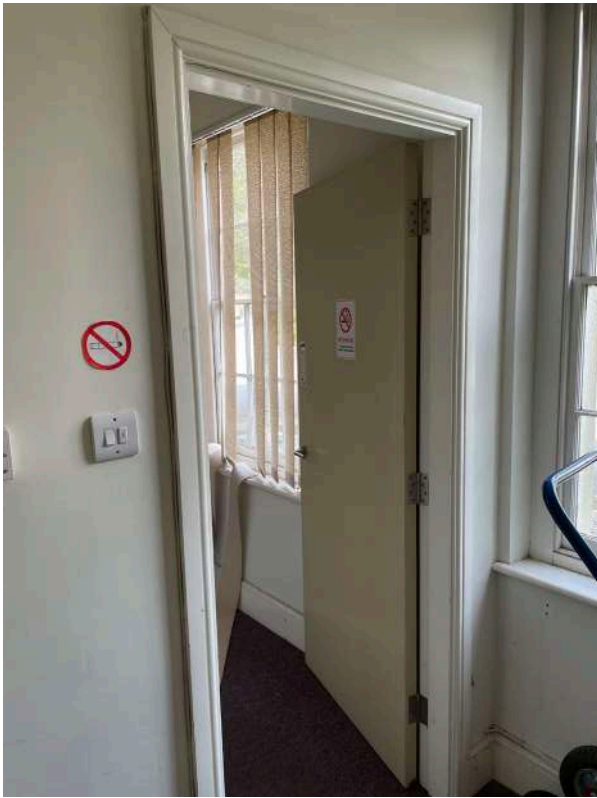
Q1.5 - Modern door and architrave to BFS office (20)
