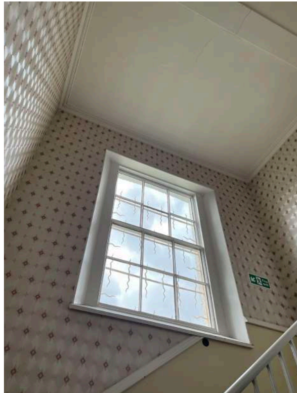
R9 - Sash window on stairwell (1B)
