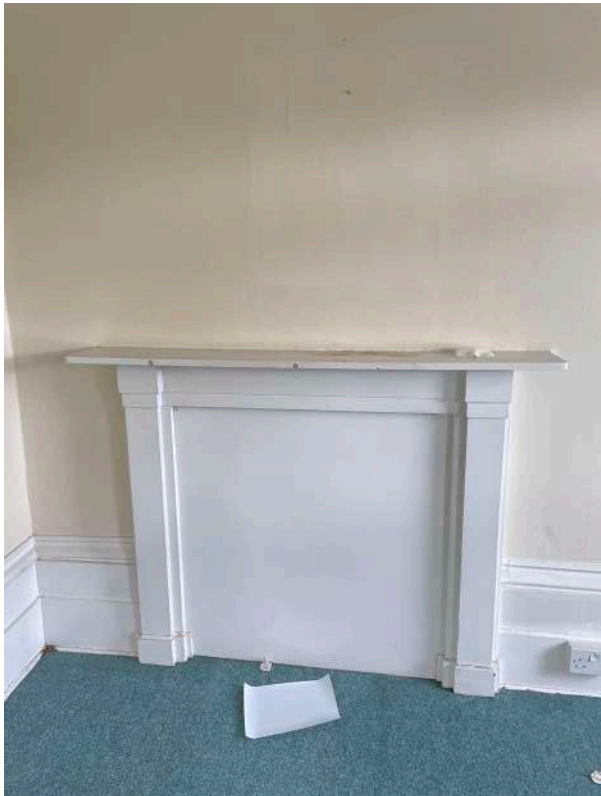
L2.8 - simply designed fireplace blocked up in office A (44)
