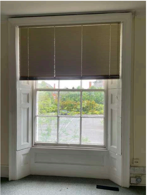
D11 - 6 over 6 sash window and shutters in Office C (14)
