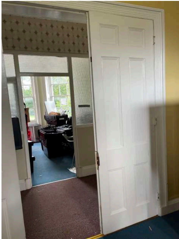
J3 - Door between in Small Ceremony room (4) and Corridor (2)
