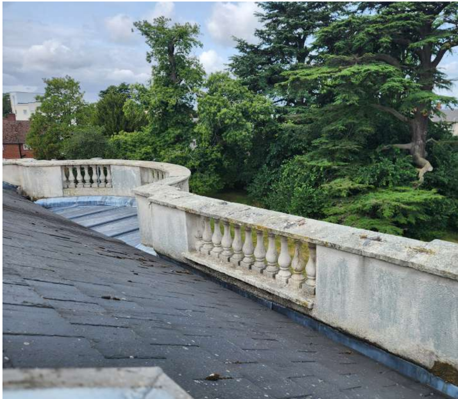
A1 - view west out of roof hatch in western storeroom (17)
