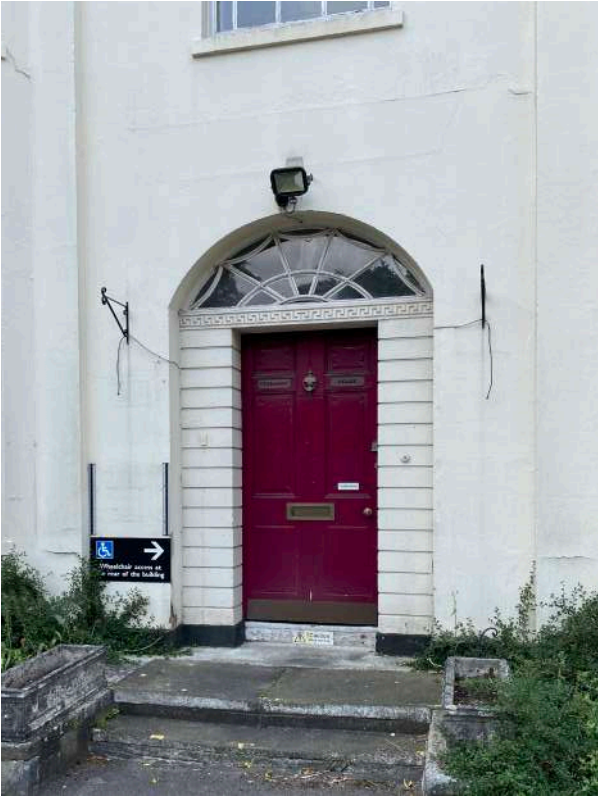
T1 - Main entrance, proposed as communal entrance to units 1-5.
