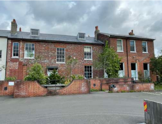
U9 - steps and ramps to rear access accompanied by raised landscaping
