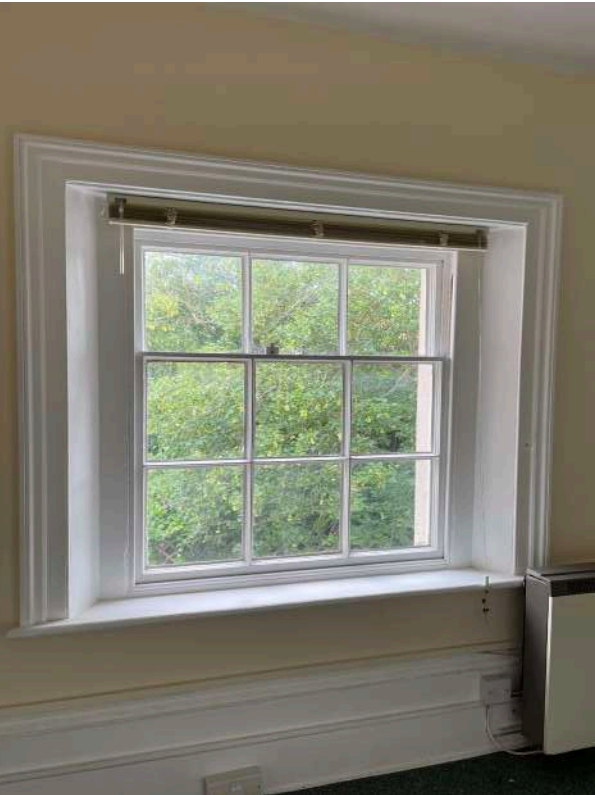
L2.2 - decorative window surround and high skirtings in Office C (47)
