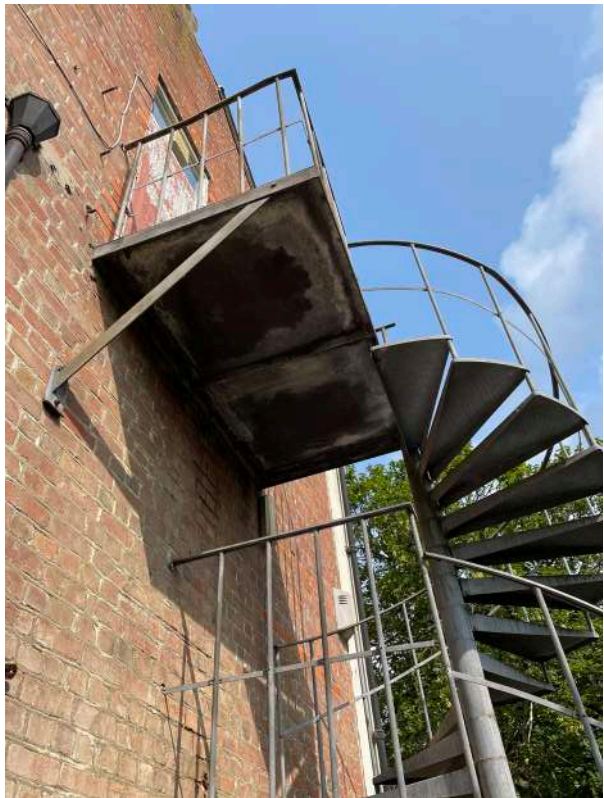
K1 - Red bricks East facade with fire escape helical metal stair
