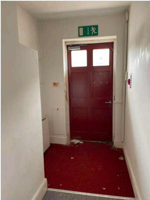
Q1.2 - modern fire door to rear elevation in corridor (19)
