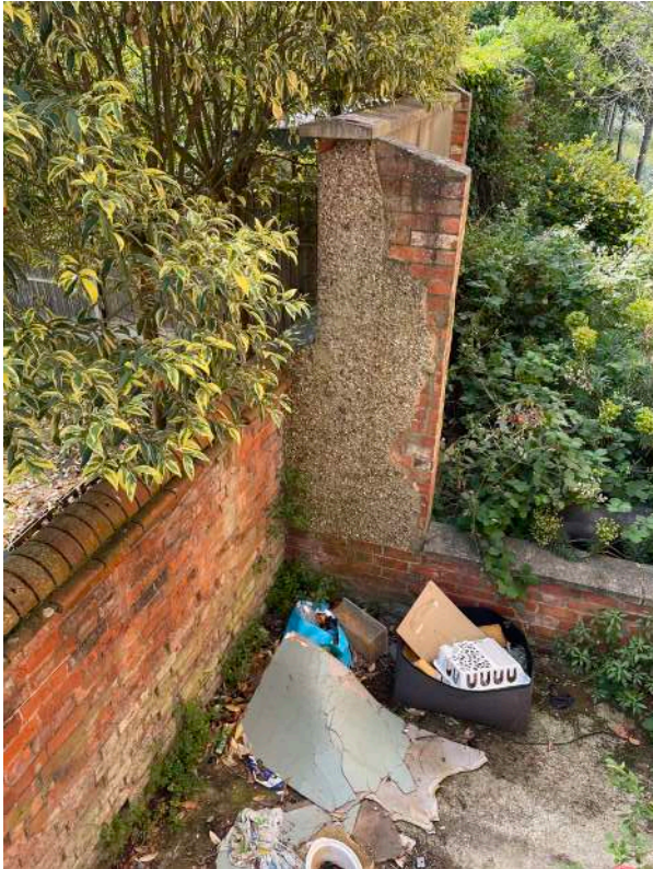
U2 - East boundary wall
