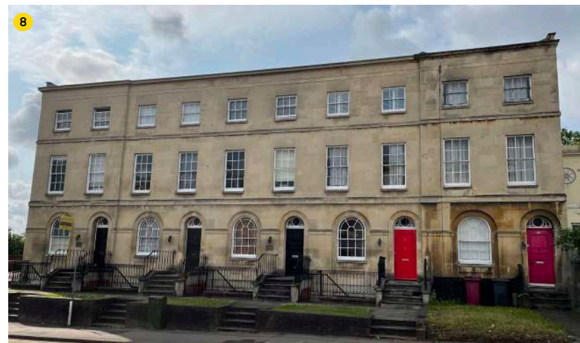
Blenheim Terrace, Bath stone terrace, Castle Street with original arched windows and fanlights
