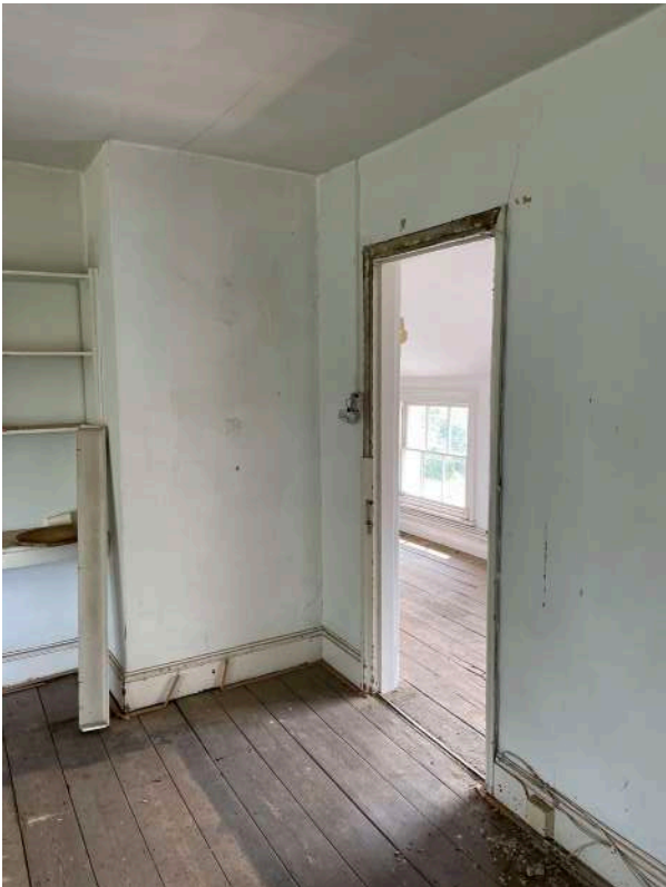
Q3.6 - door between central room (35) and kitchen (34)
