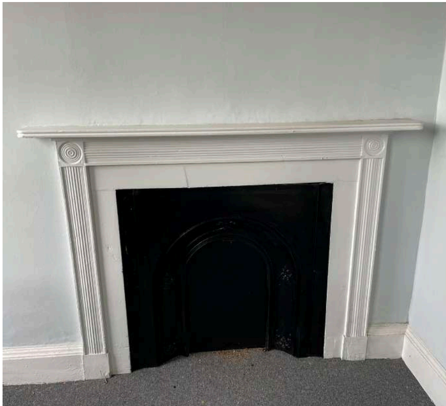
F10 - simple fire surround in Office B (12)
