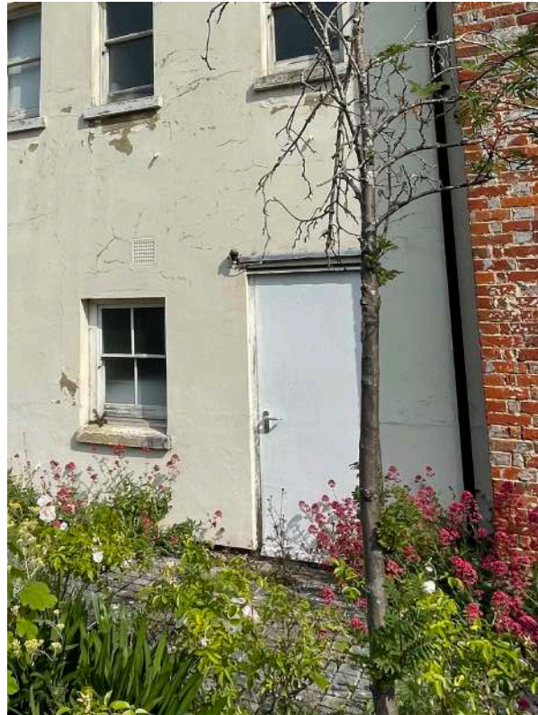
T6 - rear storage door, proposed as garden access door to unit 6.
