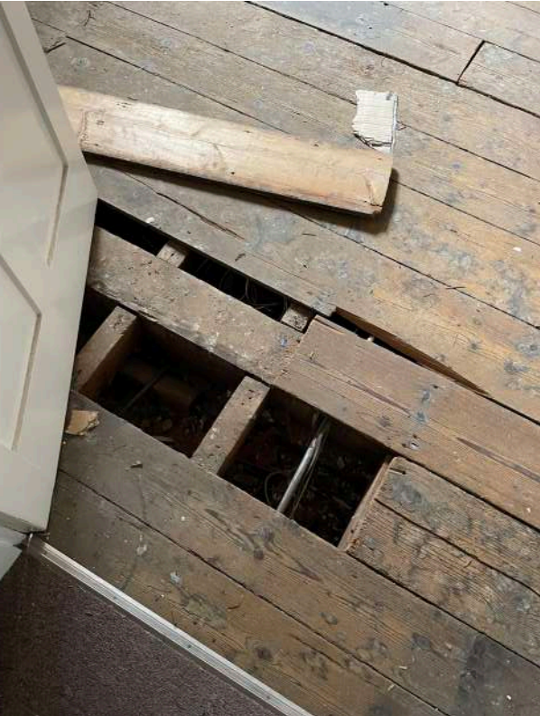
B5 - Existing flooring in eastern storeroom (18)
