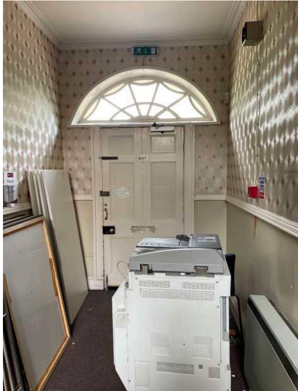
R1 - Entrance hall and Georgian entrance door with fanlight (1A)
