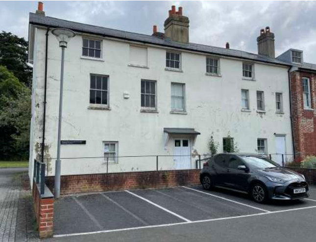
U8 - Existing parking to the southern boundary
