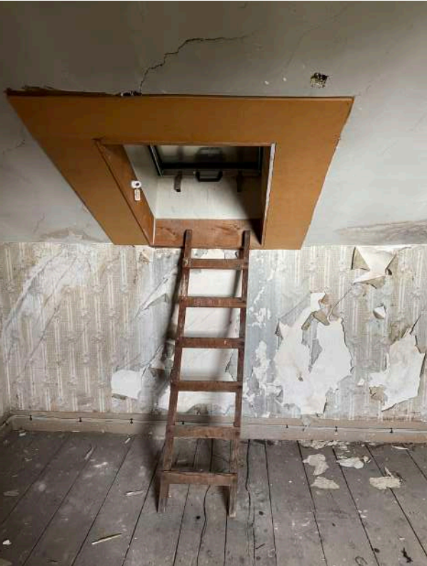
B6 - Western storeroom (17) modern access hatch with historic ladder
