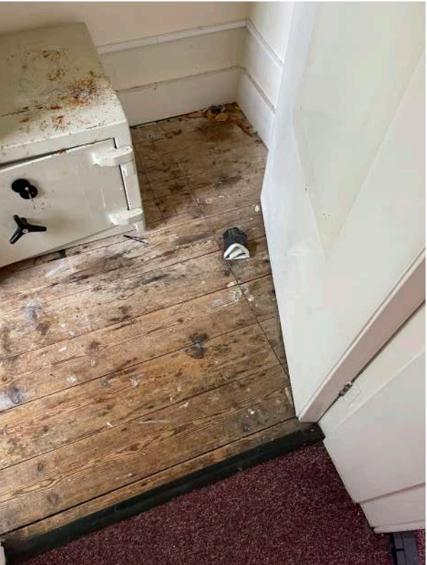
L1.6 - Floorboards in washroom (40)
