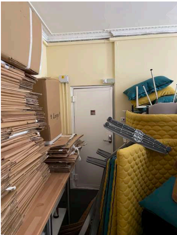
H8 - cornice and modern door in administration office (5). door to be blocked up.
