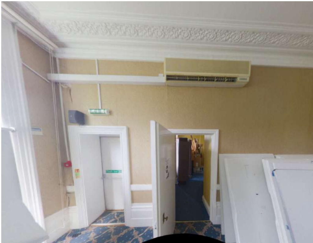
L1.9 - Wall between large ceremony room (41) and small ceremony room (4) with modern services and fire doors, and historic skirting and coving
