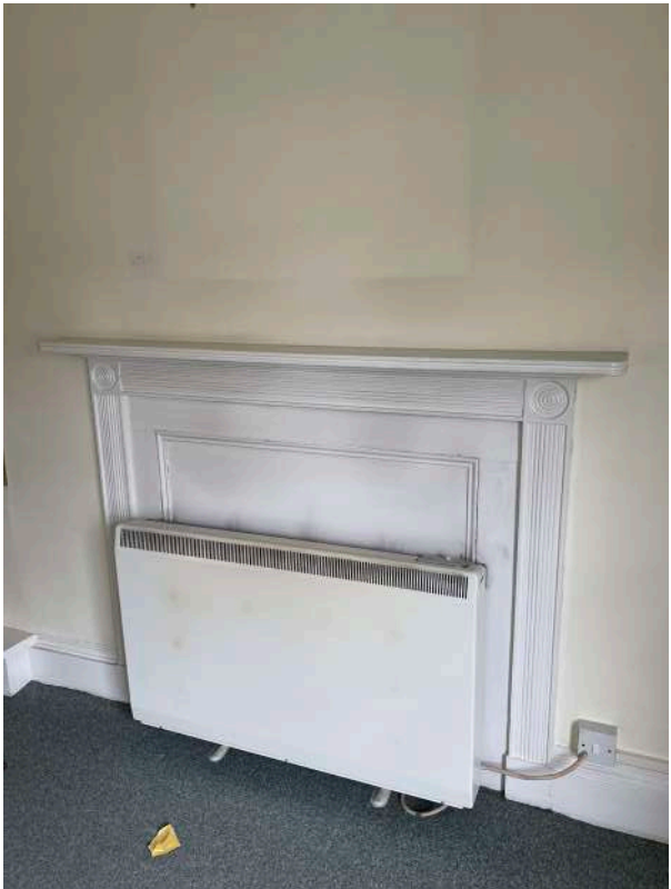
D8 - Modern radiator over closed-off fire surround in Office C (14)
