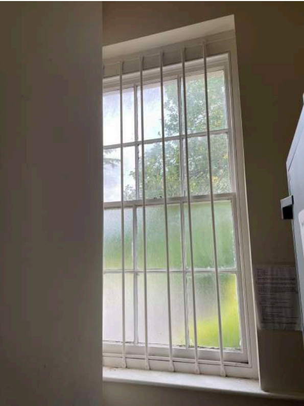
L1.4 - Timber sash window and metal bars in washroom (40)
