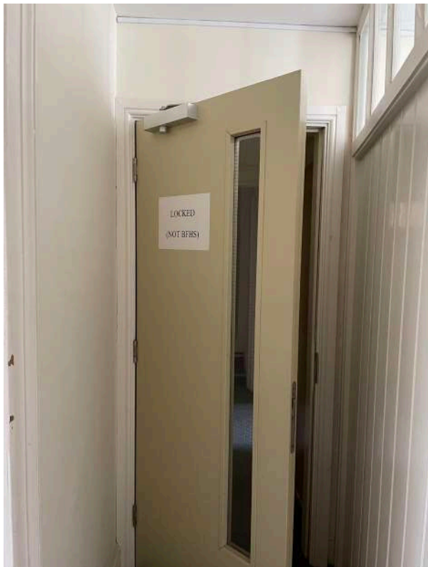
02.2 modern door between modern corridor (11) and corridor (25)
