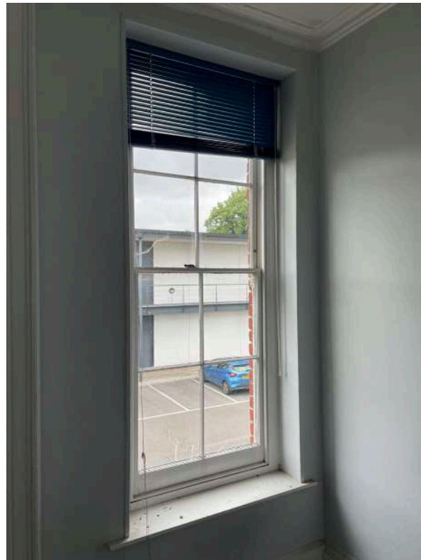
F6 - non original sash window in Office B (12)
