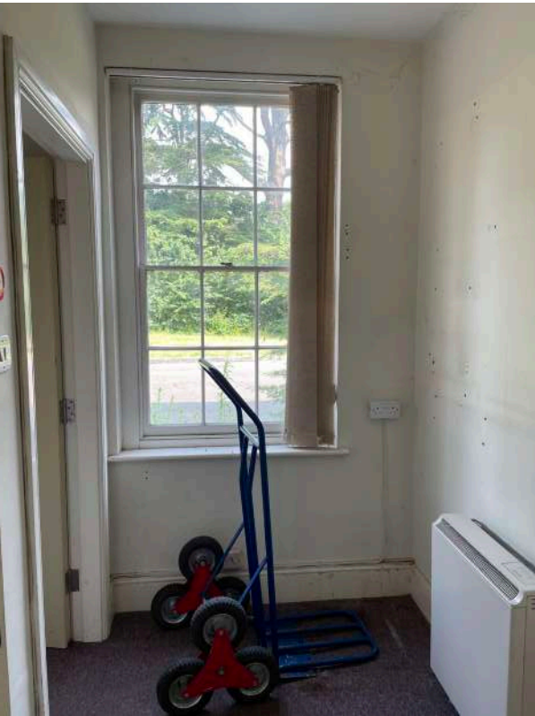
Q1.3 - window, architrave and heater in room between corridor (19) and BFS office (20)
