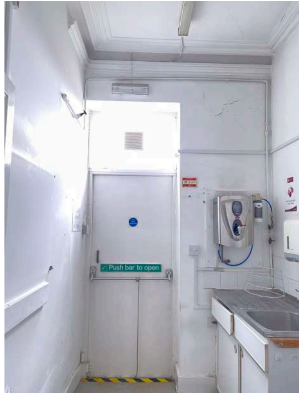
L2.5 - Kitchen and modern fire escape door to external fire escape helical stair
