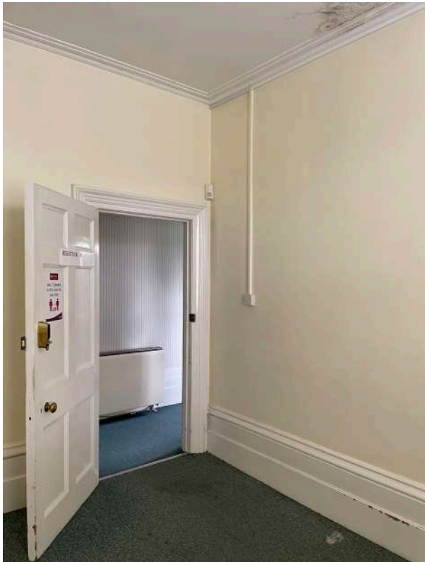
L2.9 - two types of cornice in Office B (43) suggests modern partition
