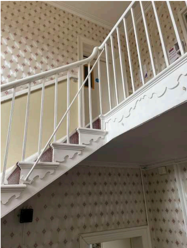
R10 - decorative stair stringer to grand staircase (1B)
