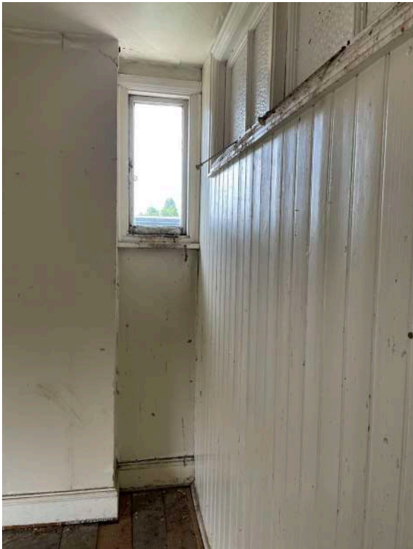
Q3.3 - small single window between chimney breast and partition in rear west room (37)
