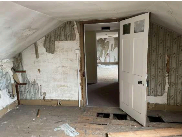
B9 - Eastern storeroom (18) door looking into attic landing (16)
