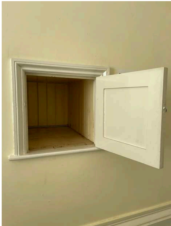
L2.13 - Dumb-waiter fixed in position with working hatch in office B (43)
