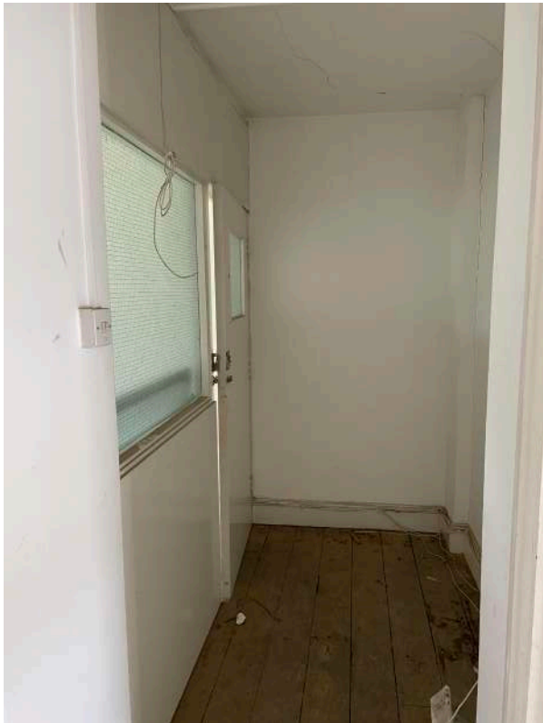
03.4 - modern glazed partition between landing (30) and corridor (32)
