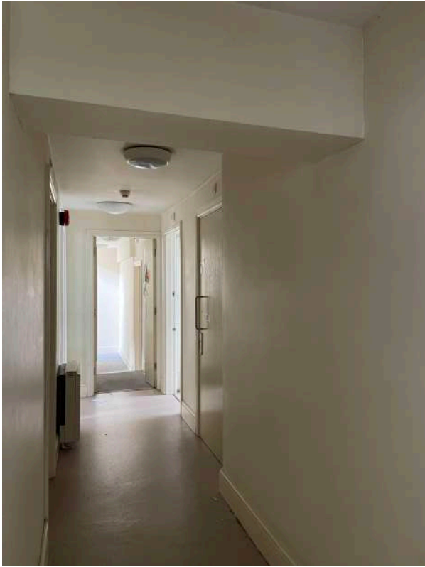
Q1.4 - downstands in modern corridor suggest modern re-configuration
