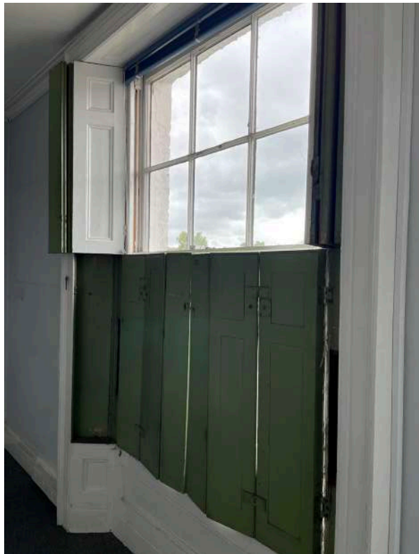
F5 - Office B (12) shutters in working condition
