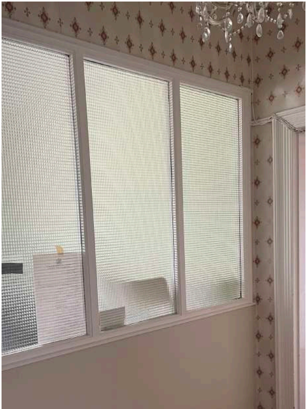
J5 - picture rail is interrupted between Corridor (2) and Deputy Office (3)
