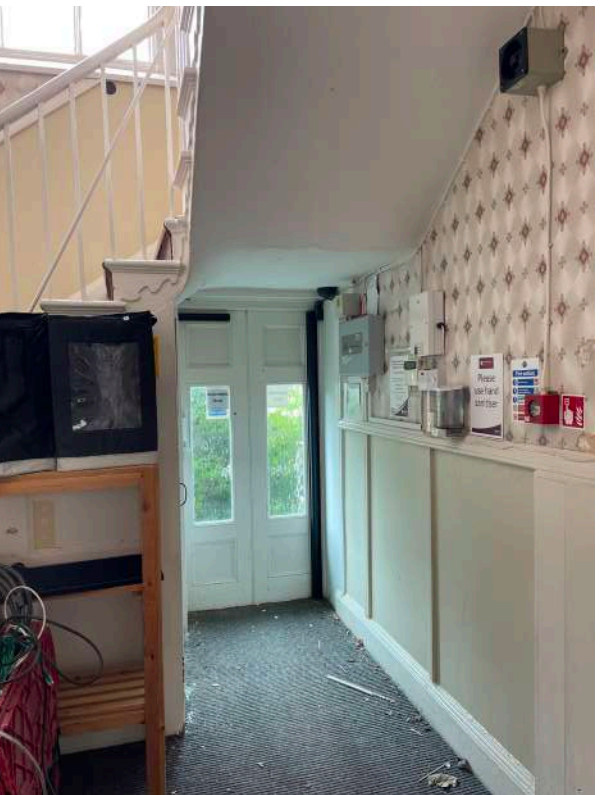
R6 - Back glazed door, Wall panelling and dado (1A)
