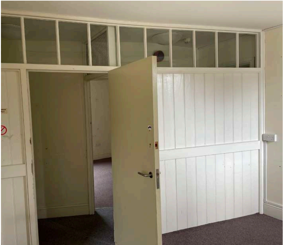
02.3 - modern partition in store room (27)
