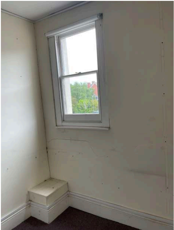
Q2.6 - Low level boxing in store room (27)
