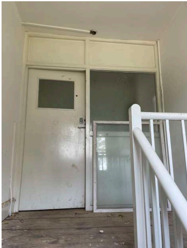
03.1 - modern glazed partition between landing (30) and corridor (32)
