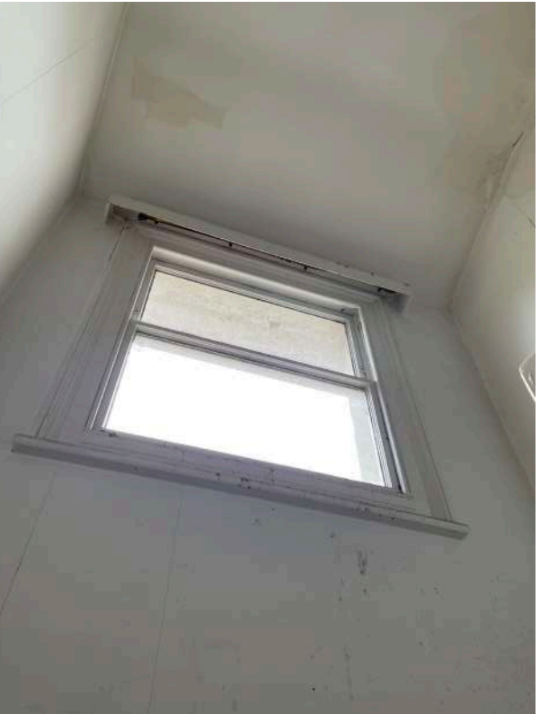
O1.4 - window in stairwell (29)
