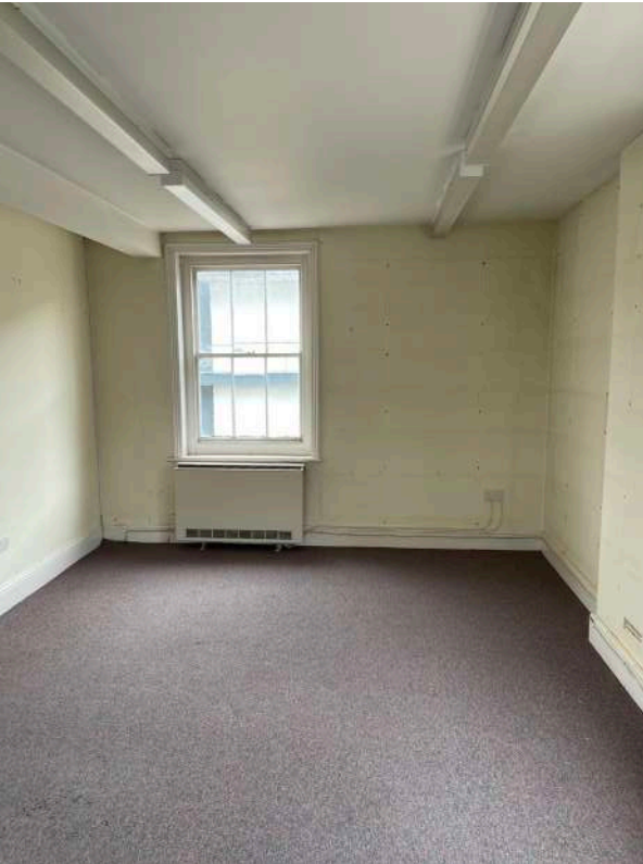
Q2.4 - series of downstands in exhibition room (26) suggest modern reconfiguration
