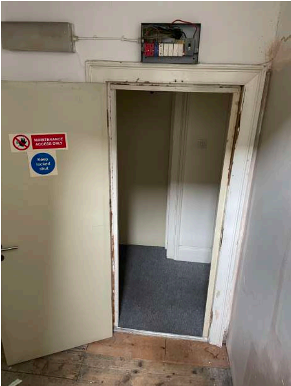
01.6 - door from stairwell (29) to modern corridor (11)
