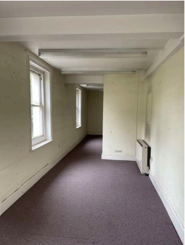
Q2.5 - series of downstands in exhibition room (26) suggest modern reconfiguration
