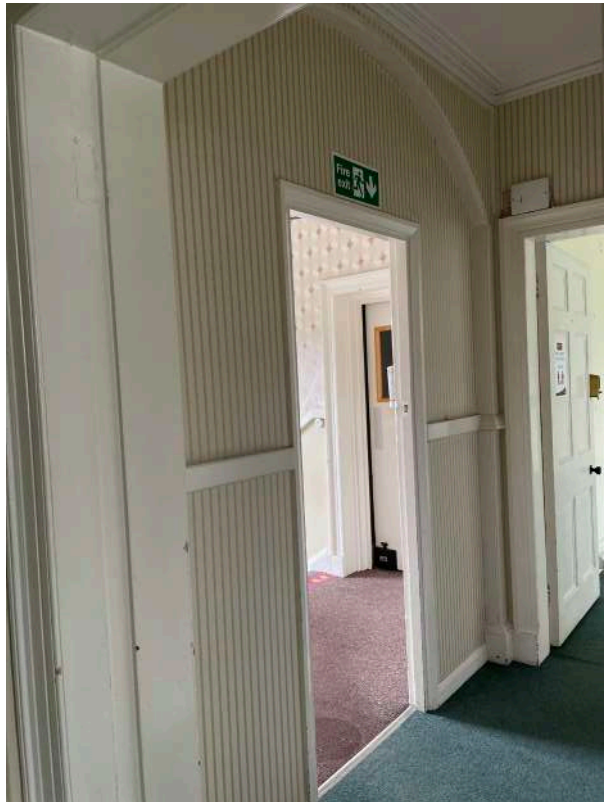
D1 - Historic archway with modern partition and fire door between stair and landing (7)
