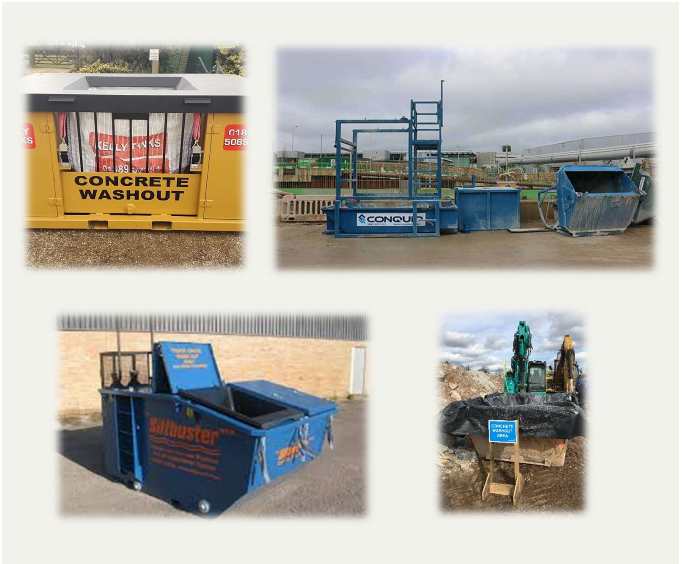
Figure 3 - Examples of Concrete Washout systems that may be utilised on site
