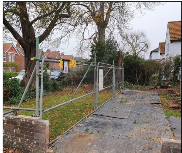
GP2: Tree protection barriers & trackmat ground protection
