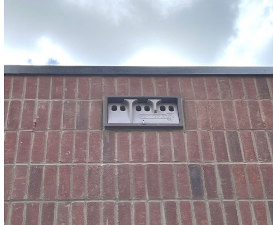
2. Installed Schwegler 1SP Sparrow Terrace
