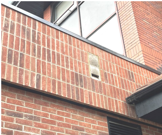
3. Installed Schwegler 1FR Bat Tube
