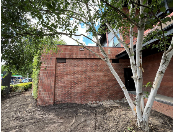
1. Location of installed bat and bird boxes
