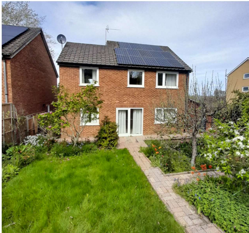
Looking towards the rear (southerly facing) elevation
