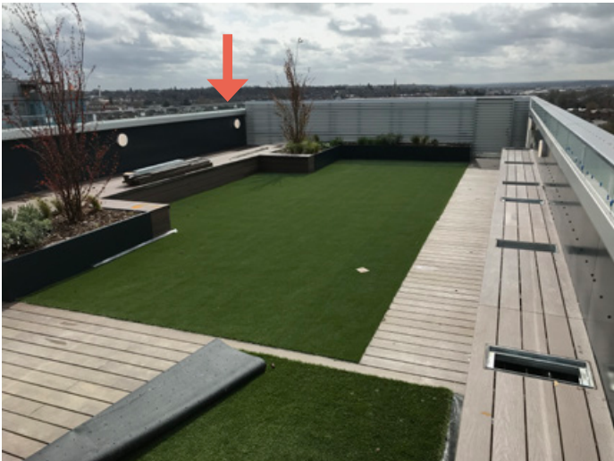
Above: Aerial view of proposed location of stair, indicated by red arrow. (Photograph taken during construction). Below: Amenity space at roof level. Location of top of stair indicated by arrow.
