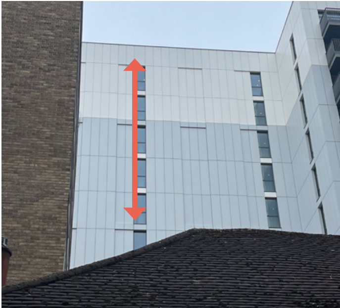
Above: Photograph of existing elevation from proposed position of the stair. Below: Photograph of the rear elevation of Plot F from the east side of Merchants Place. Stairs location highlighted by the arrow.
