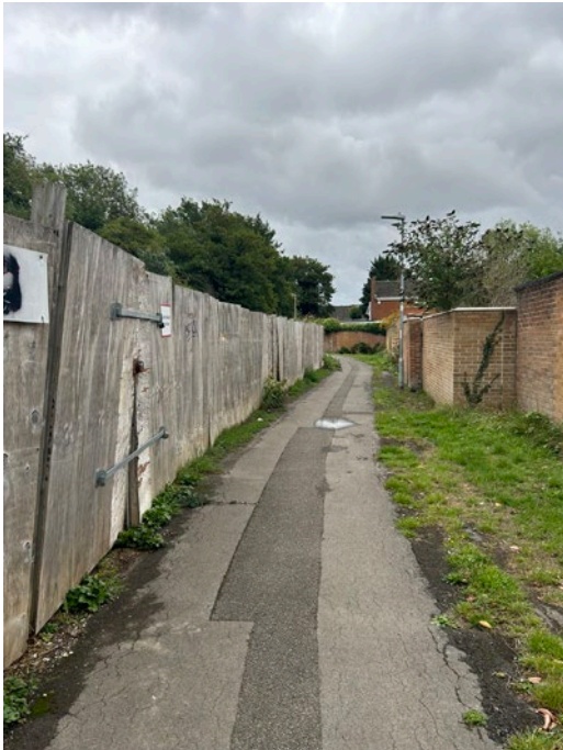
Existing pedestrian access
