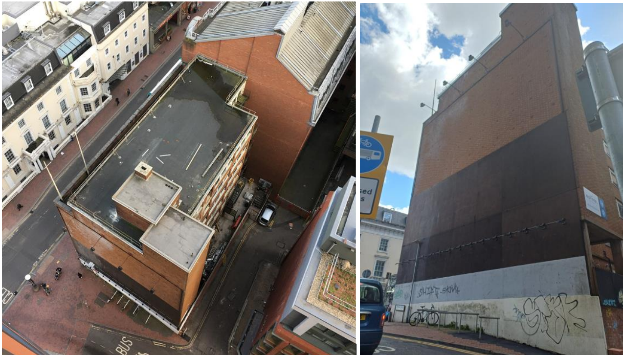
View from within Thames Tower (from 2019) and street level (April 2026)
