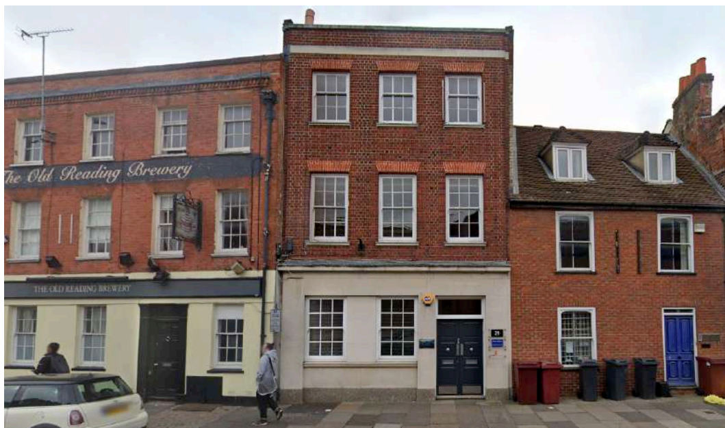
Figure 2 – View of the access from Castle Street (North)
