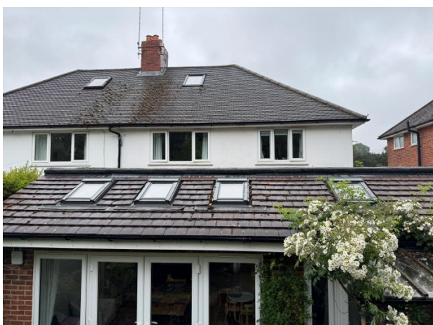
Photograph 3. The south-western elevation of the building and adjacent property.
