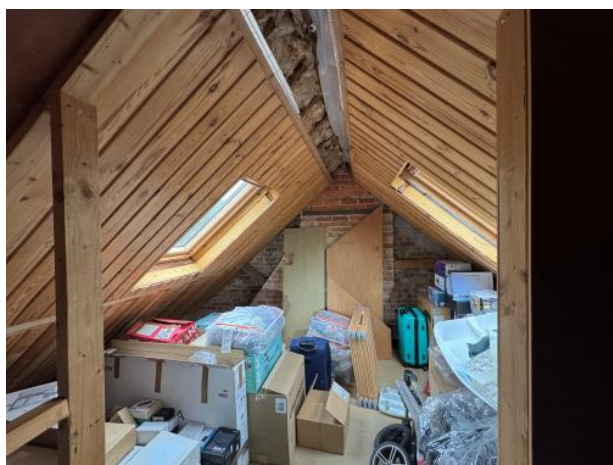
Photograph 6. The loft space within the building.
