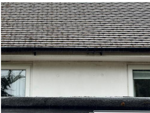
Photograph 5. Detail of the tight fitting eaves.
