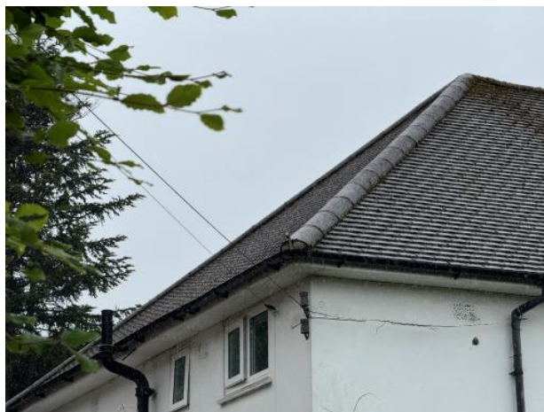
Photograph 2. The south-eastern elevation of the building.
