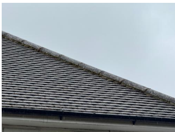
Photograph 4. Detail of the tight fitting roof tiles and ridge tiles.
