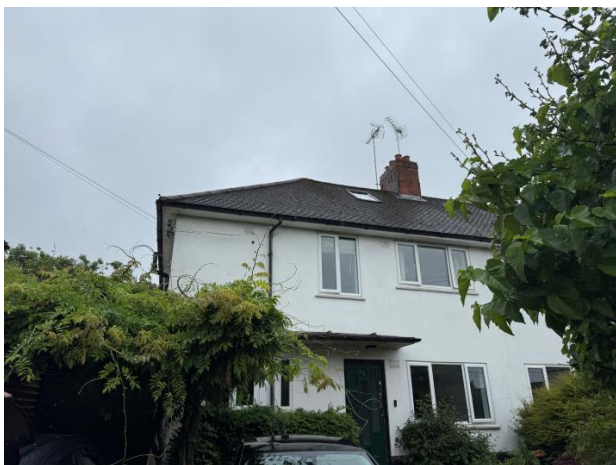
Photograph 1. The north-eastern elevation of the building.
