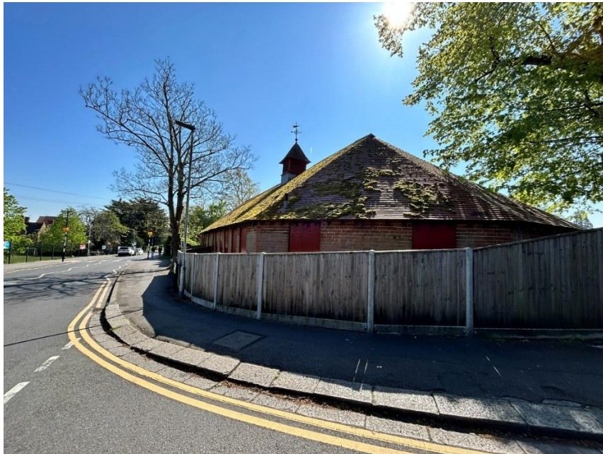
Figure 5: Boundary fence to No 11 Elmhurst Road
