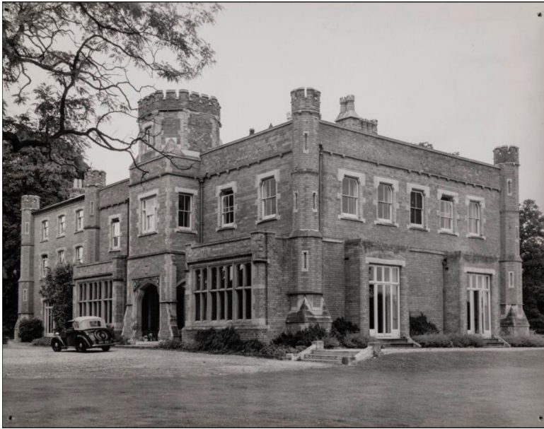
Figure 3: Park House in the early 20 th century 13 .
