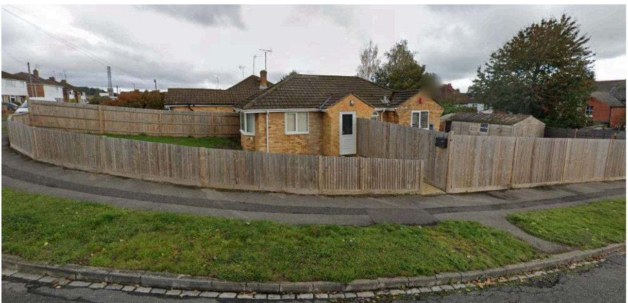
Figure 2 – View of the house from Amblecote Road (South)
