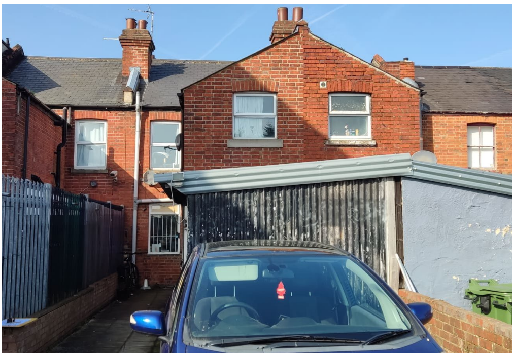
Fig 4. Rear view of Tilehurst cobbler including the corrugated metal shed originally used as a cold store
