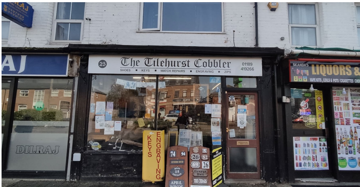
Fig 3. Front façade of Tilehurst Cobbler as seen from School Road
