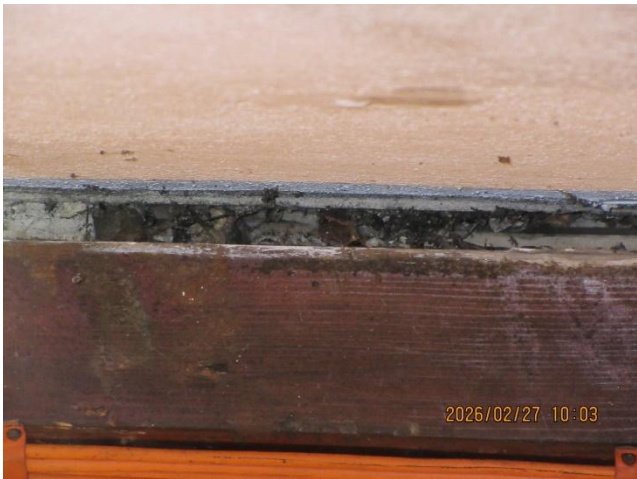
Photos 7 and 8– Bat droppings found inside the north chapel and gap between the timber frame and the eastern end wall
