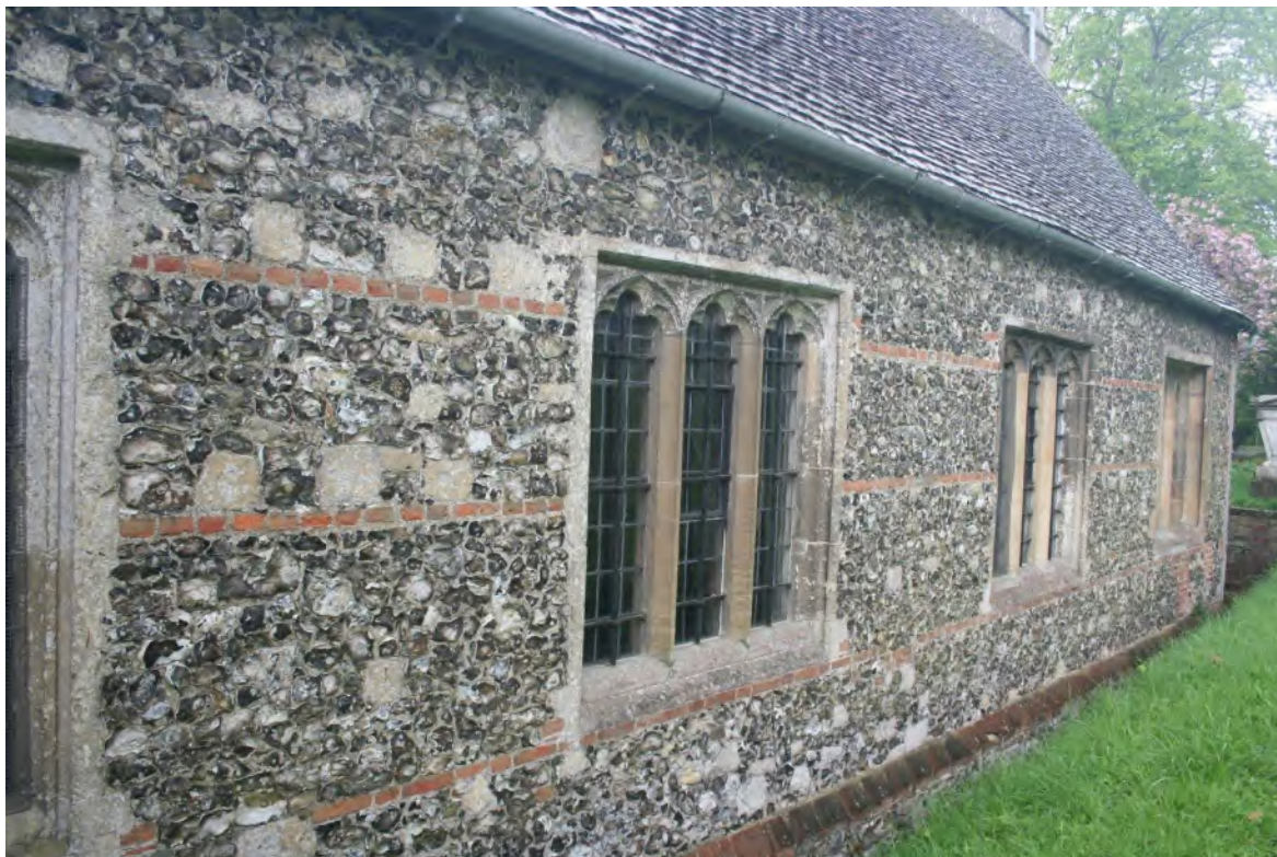
Fig 7: North aisle. The possible Norman stone is just visible below the third window from the west, just above the plinth.
