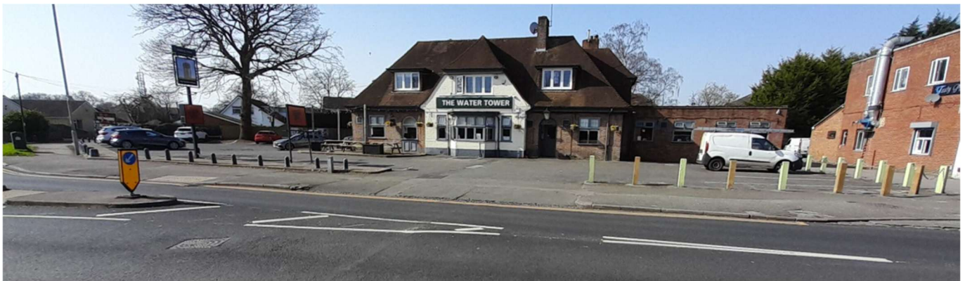
Front elevation looking from Park Lane
