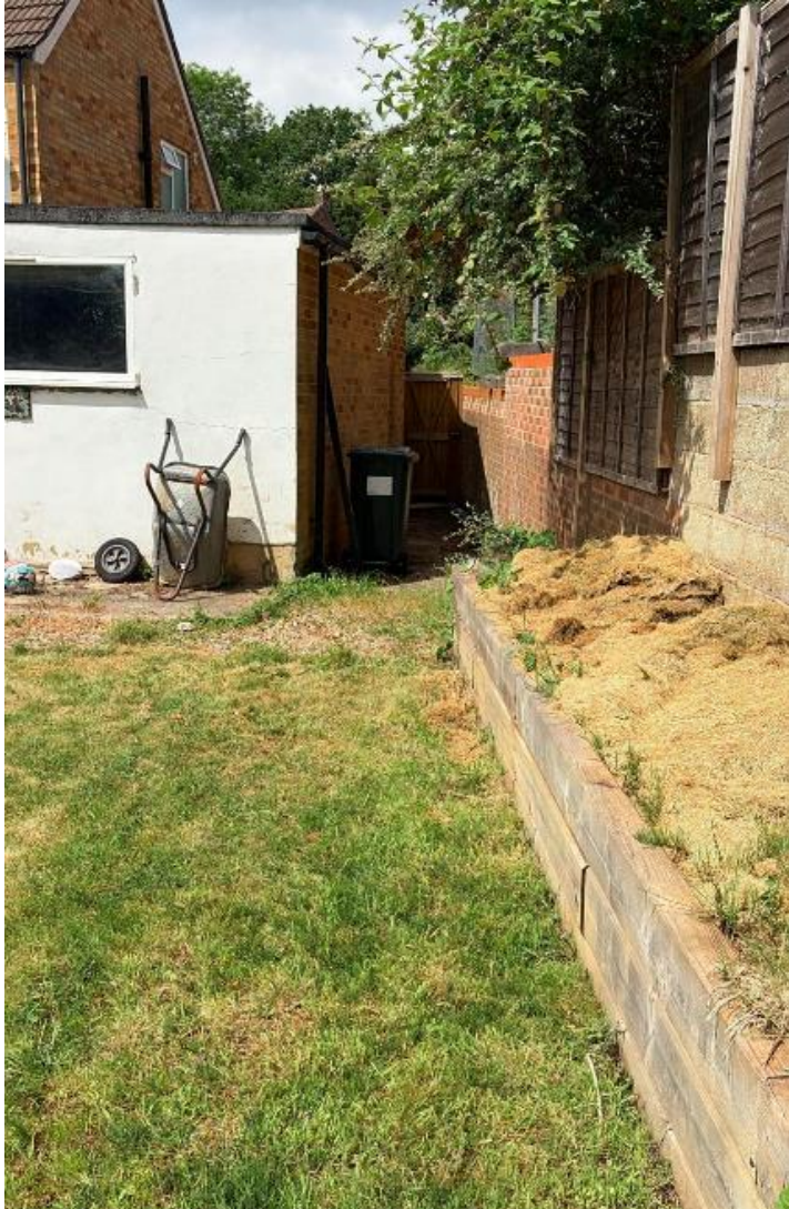
Side alleyway providing access to the rear garden, including retaining wall and boundary fencing.
