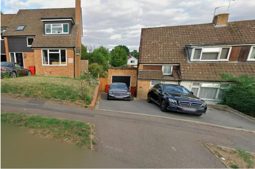
Front elevation of the house showing the existing garage and retaining wall.
