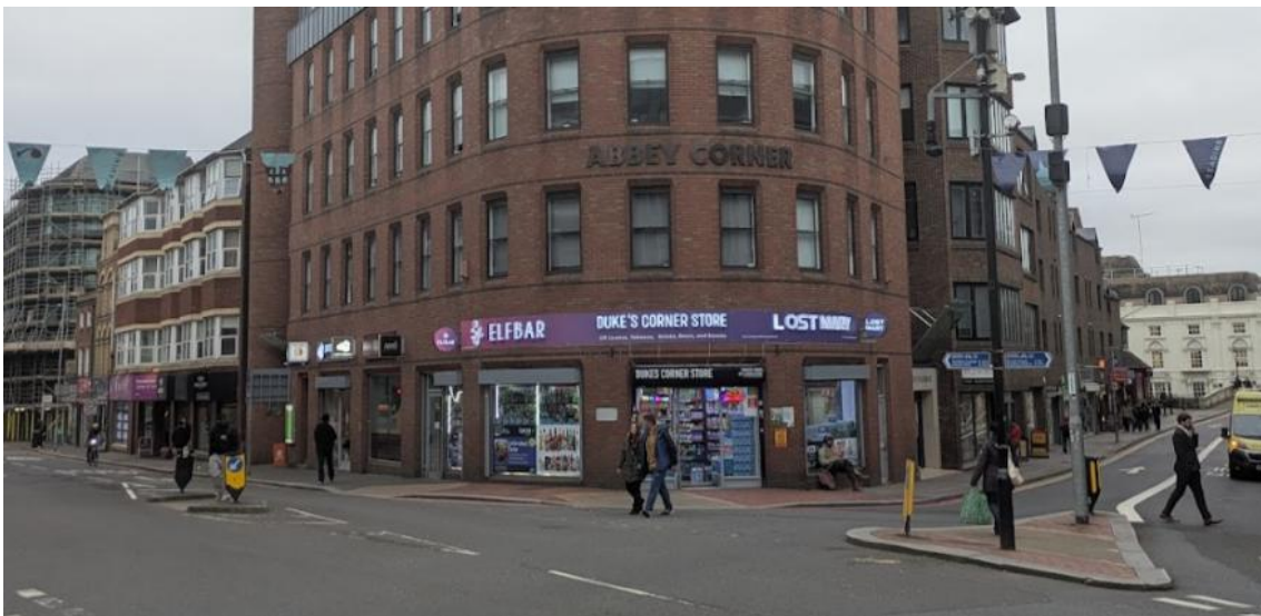
Figure 1 Photo of the application site taken by the case officer in April 2026.
