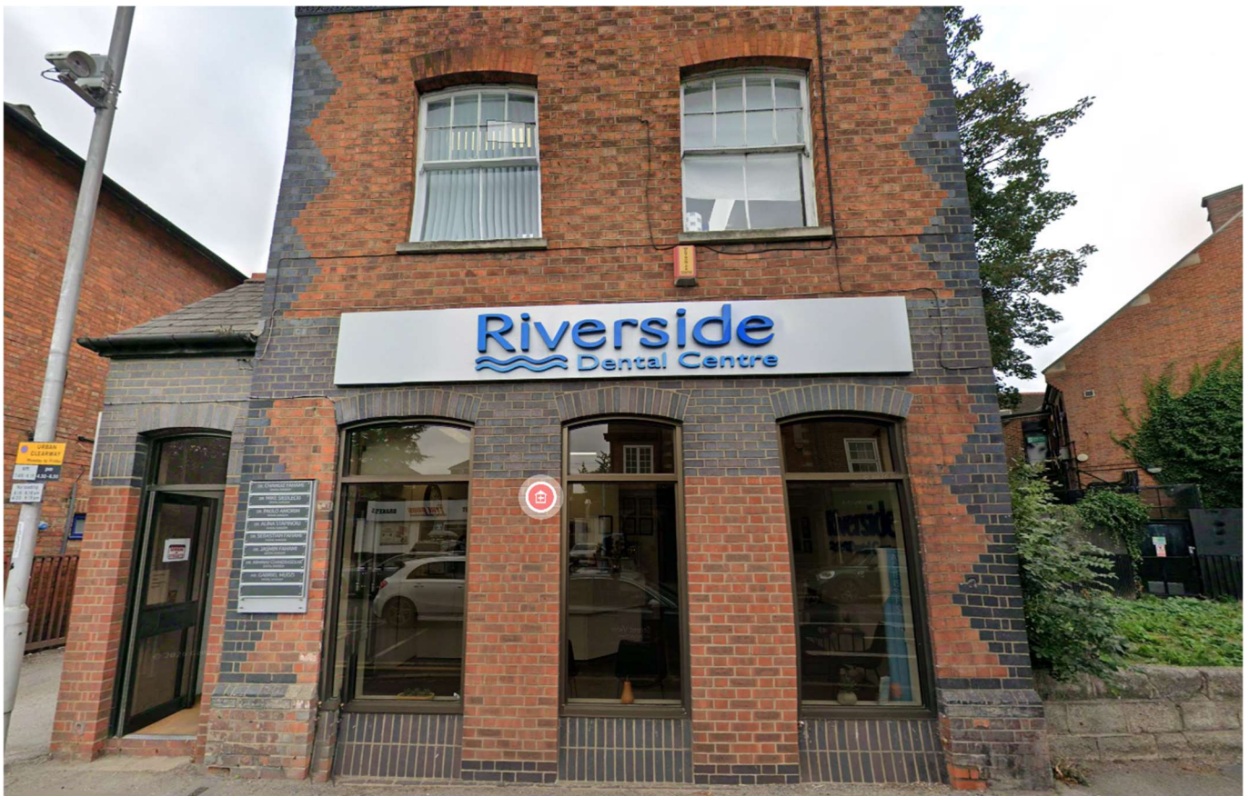
Front – easterly facing elevation.
