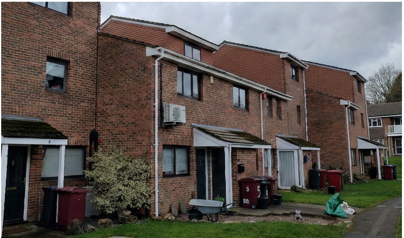
Above View of front facade showing the current location of the AC unit
