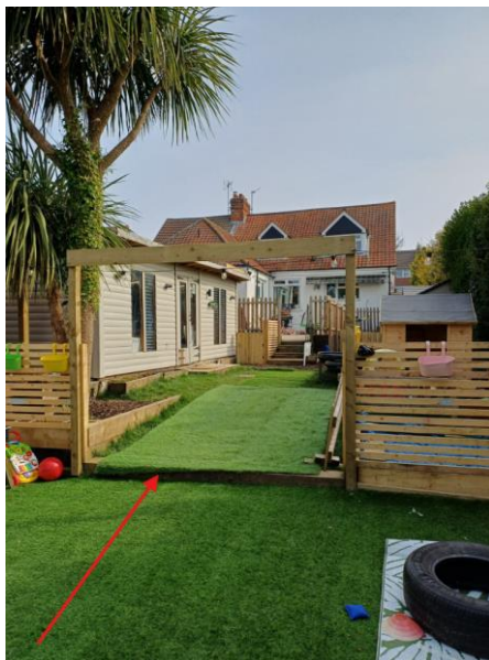
Site Visit Photographs – clear artificial grass
