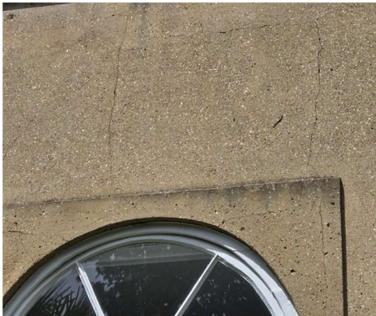
Photos showing cracking and legacy alarm box that will be removed
