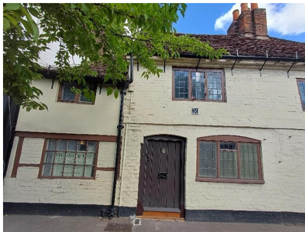
View from the front of 6 Church Street, taken 08/07/2025.
