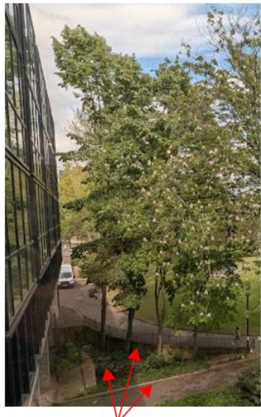
Wall and fence with established planting and kerb line
