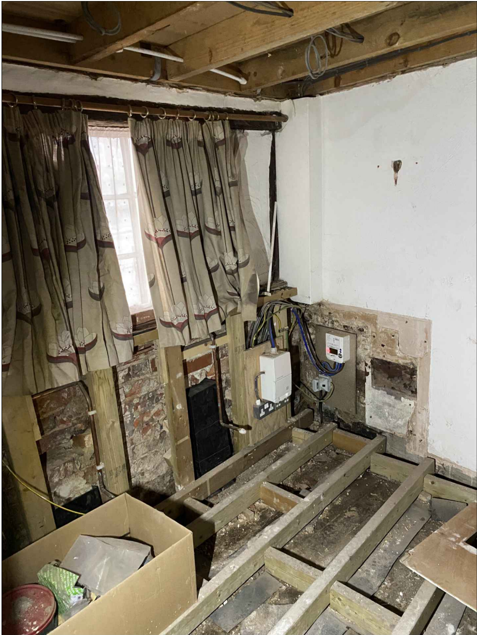
The existing mid-C20 softwood Snug ceiling & Dressing Room floor joists (top of image) of low significance in-situ - NTS
