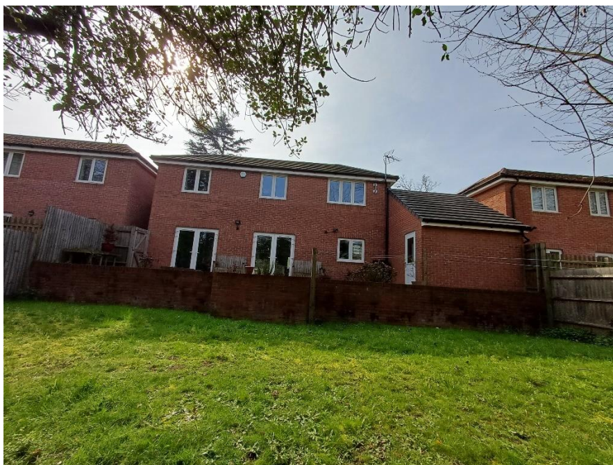
Rear View of 22 Wellswood Garden, taken 20/03/2026
