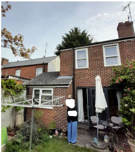
Existing rear elevation detached from neighbouring terraced properties
