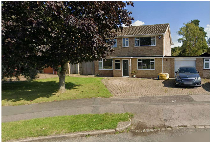
Front elevation of application site (Google Maps)
