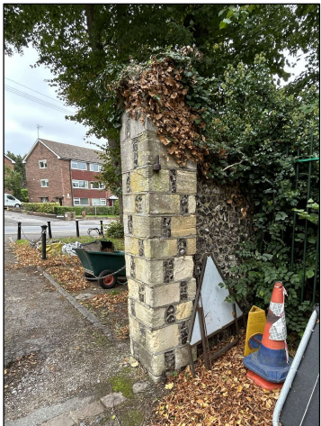
05 Stable Gate Piers NTS
