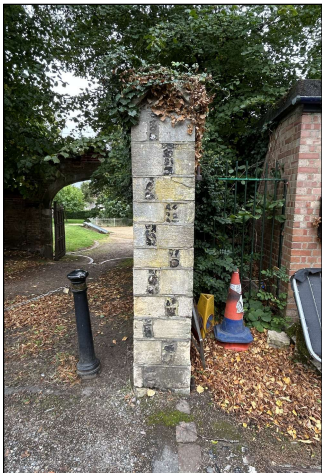
04 Stable Gate Piers NTS
