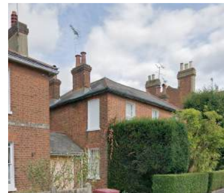
SIDE BLOCKOUT WINDOWS
