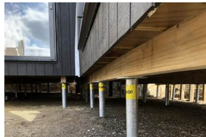
EXAMPLE OF BUILDING ON GROUND SCREWS
