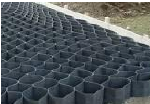
Fig 4 shows an example of Cellular Confinement System (CCS) during installation
