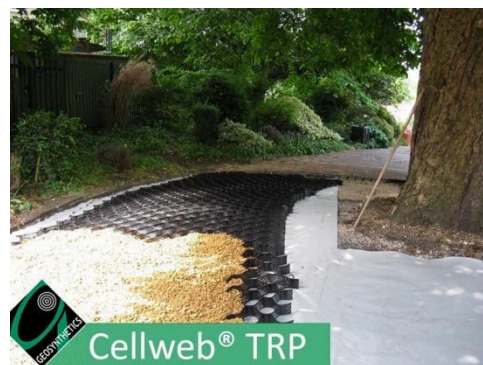
Fig 5 Shows Cellweb geo textile membrane being infilled close to a tree stem
