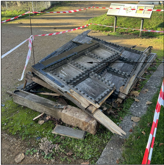
02 Damaged Main Entrance Gates and Bollard NTS
