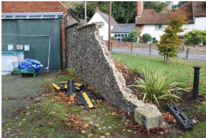
Stable Block – east boundary wall and gate piers after vehicle impact damage
