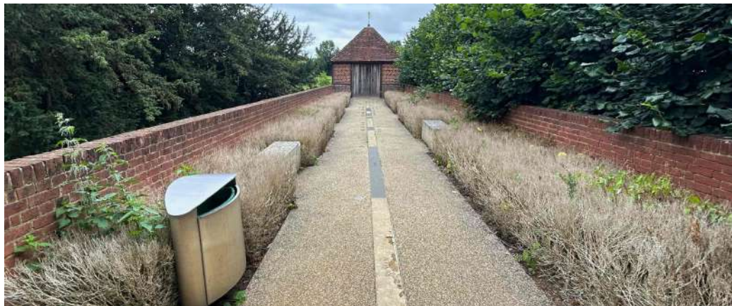
Raised Walk (Causeway) – view of the top of the Causeway looking south towards the Gazebo and river
