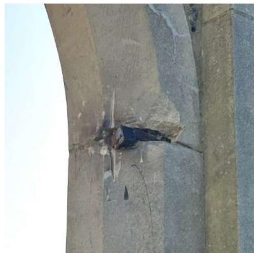
Eastern boundary (screen) wall (part): replacement double vehicular gates – destroyed gates and damage to gate hinge pins.
