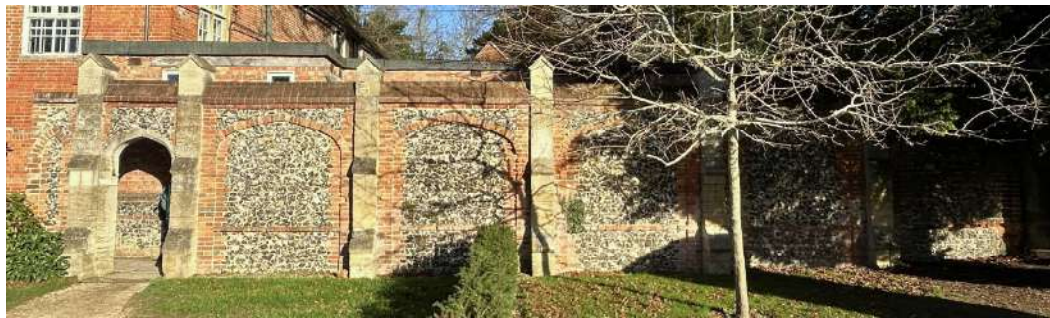
Courtyard Forecourt North Wall south face viewed from the main Caversham Court east entrance courtyard.
