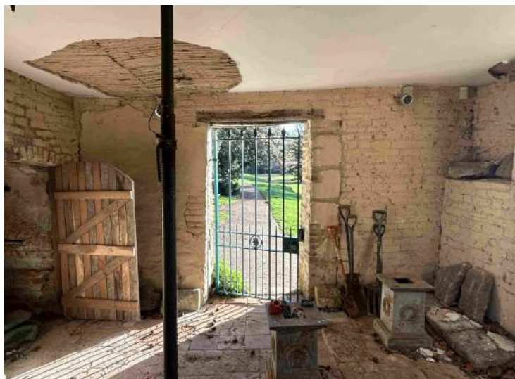
Gazebo – lower chamber – view looking at the east
