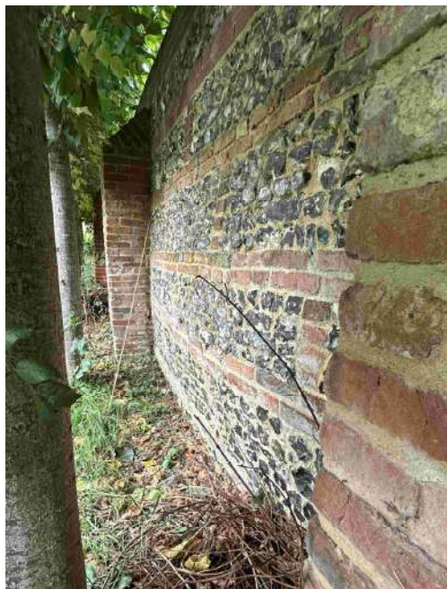
Raised Walk (Causeway) – west facing retaining wall towards the south end. Views showing 'bulging brick and flintwork panel.
