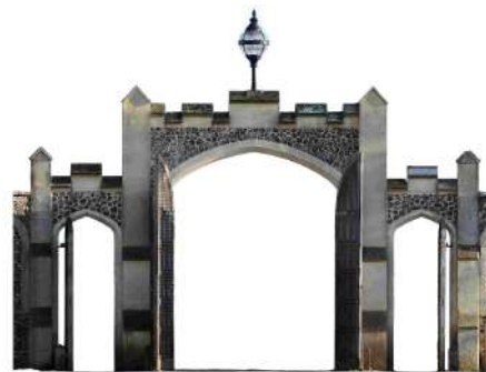
Eastern boundary (screen) wall (part): inner west elevation facing Caversham Court courtyard
