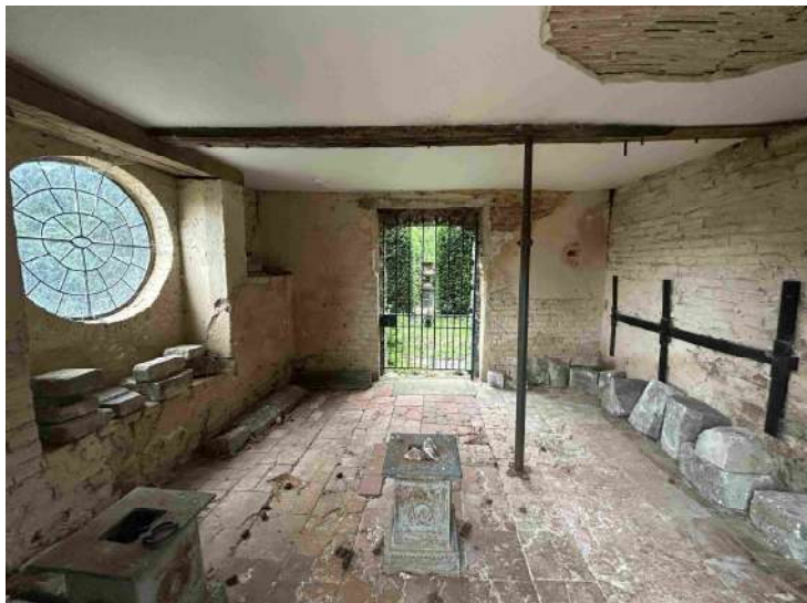
Gazebo – lower chamber – view looking at the west
