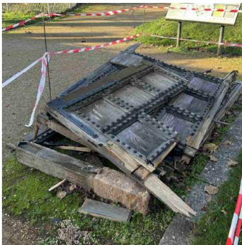
Eastern boundary (screen) wall (part): replacement double vehicular gates – destroyed gates and damage to gate hinge pins.
