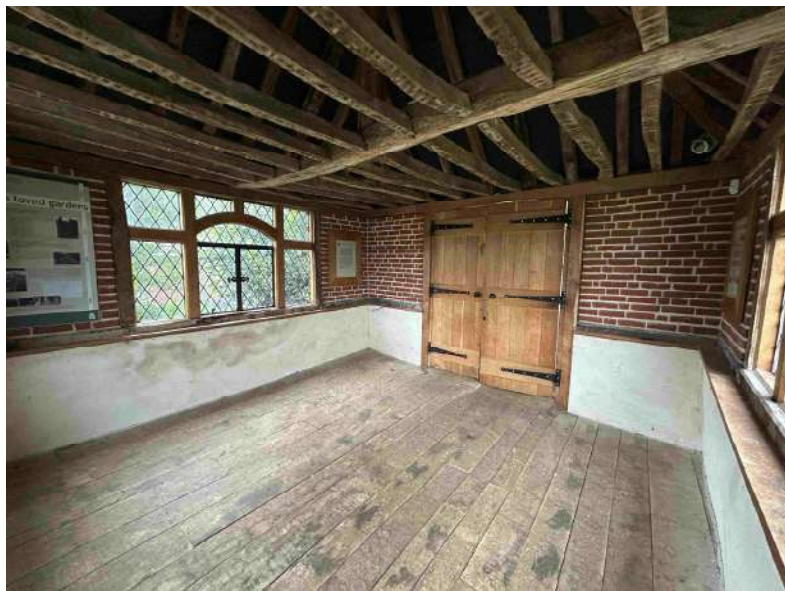
Gazebo – upper viewing chamber – view looking at the north and west walls
