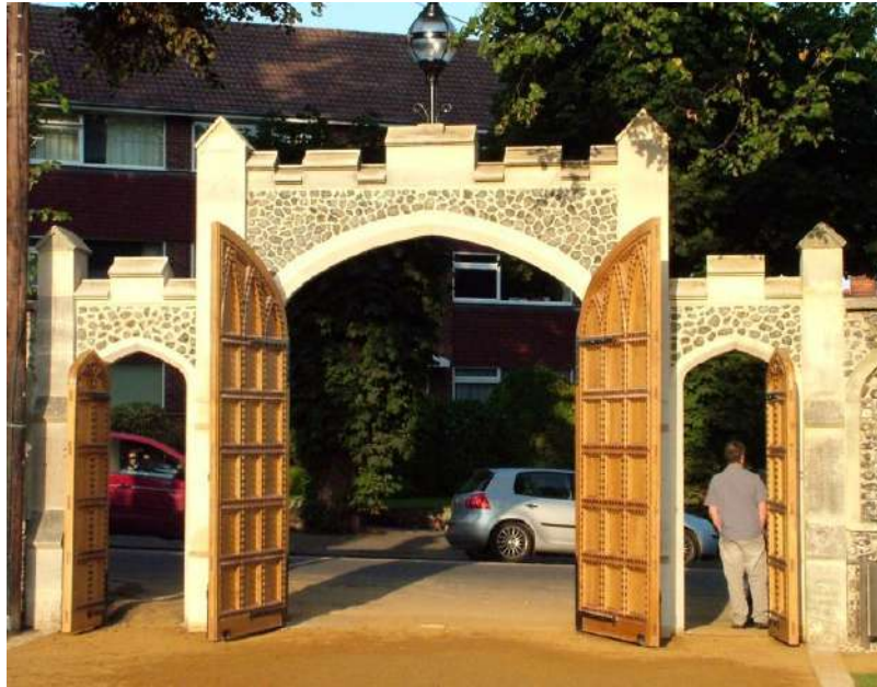
Eastern boundary (screen) wall (part): replacement double vehicular gates fitted in 2008.
