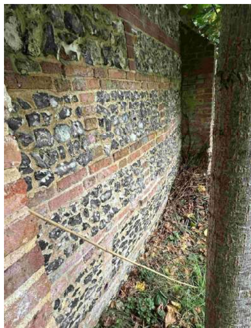
Raised Walk (Causeway) – west facing retaining wall towards the south end. Views showing 'bulging brick and flintwork panel.
