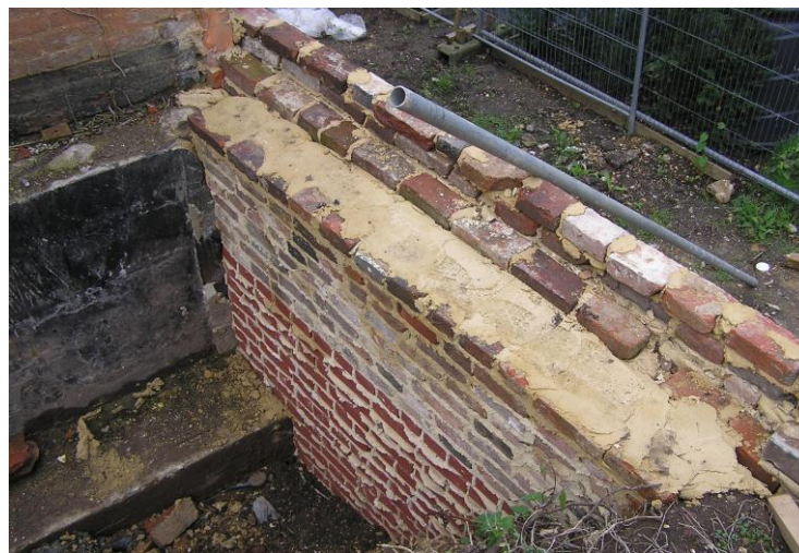
Fig. 3.10 Causeway, rear of west wall at south end, first bay adjacent to Gazebo during restoration work in 2008
