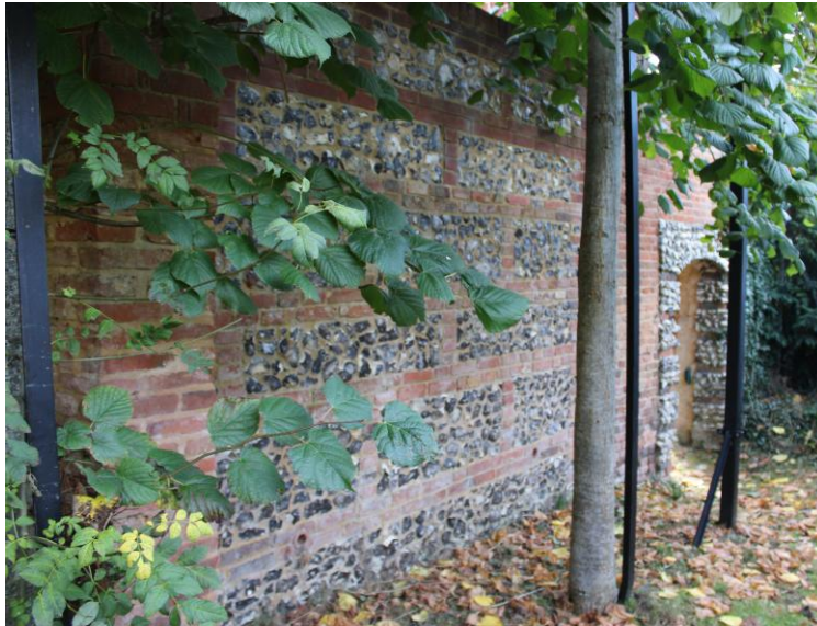
Fig. 4.1 West wall Bay 1
