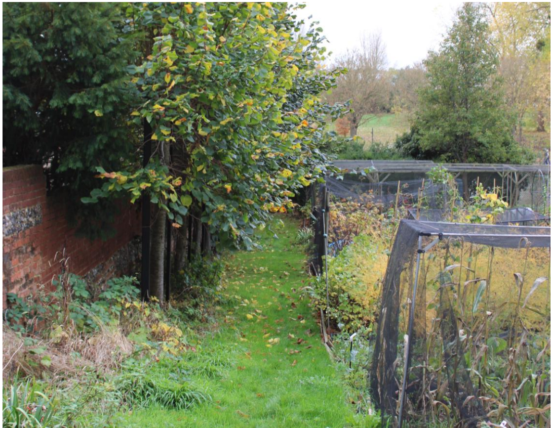
Fig. 3.5 Causeway, west wall elevation looking south
