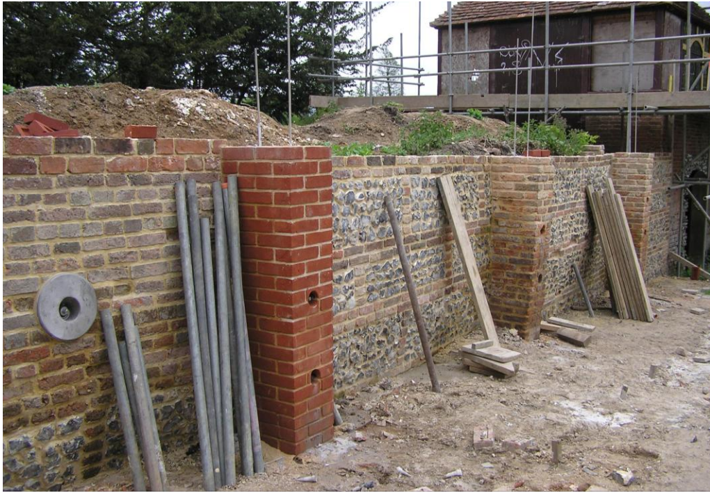
Fig. 3.9 Causeway, west wall at south end during restoration work in 2008
