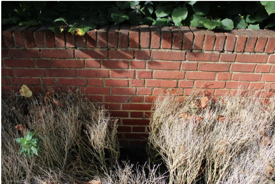
Fig. 4.11 West wall parapet and planting bed at Bay 2 from walkway level
