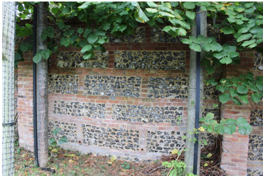
Fig. 4.2 West wall Bay 2
