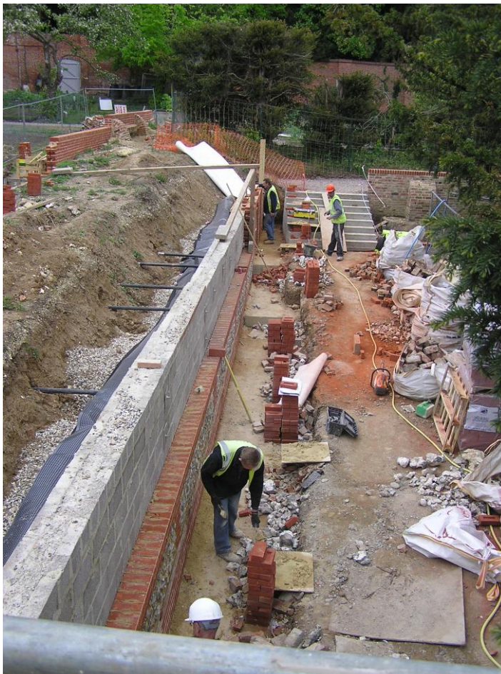
Fig. 3.8 Causeway, east wall during restoration works in 2008
