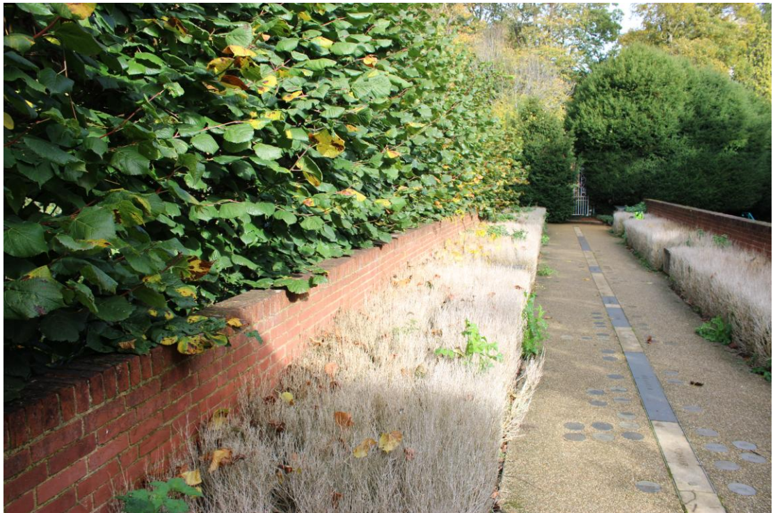
Fig. 3.7 Causeway, west wall elevation from walkway level looking north
