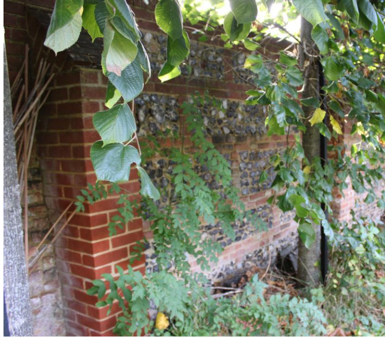
Fig. 4.7 West wall Bay 3
