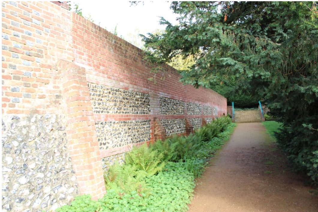
Fig. 3.2 Causeway, east wall elevation looking north
