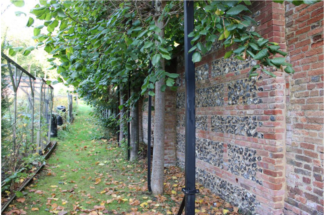
Fig. 3.4 Causeway, west wall elevation looking north
