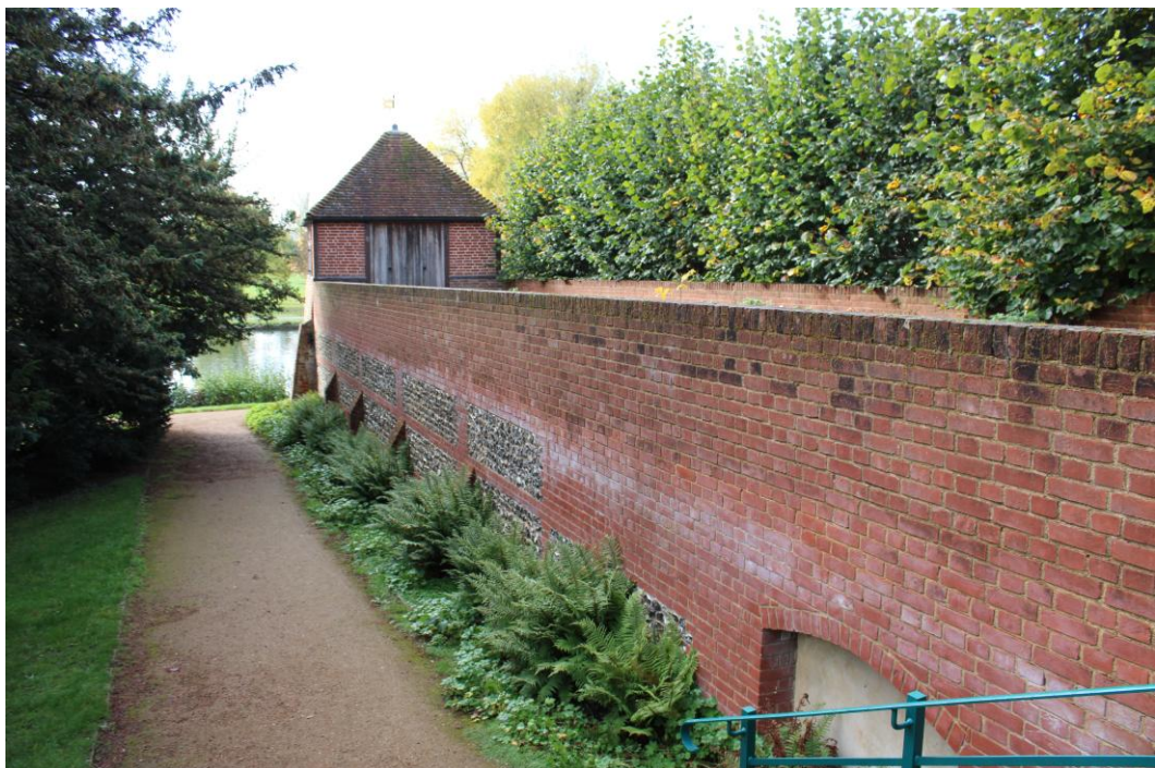
Fig. 3.3 Causeway, east wall elevation looking south (towards Gazebo)
