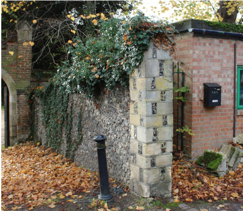
Fig. 3.6 South section of wall showing general condition of east elevation
