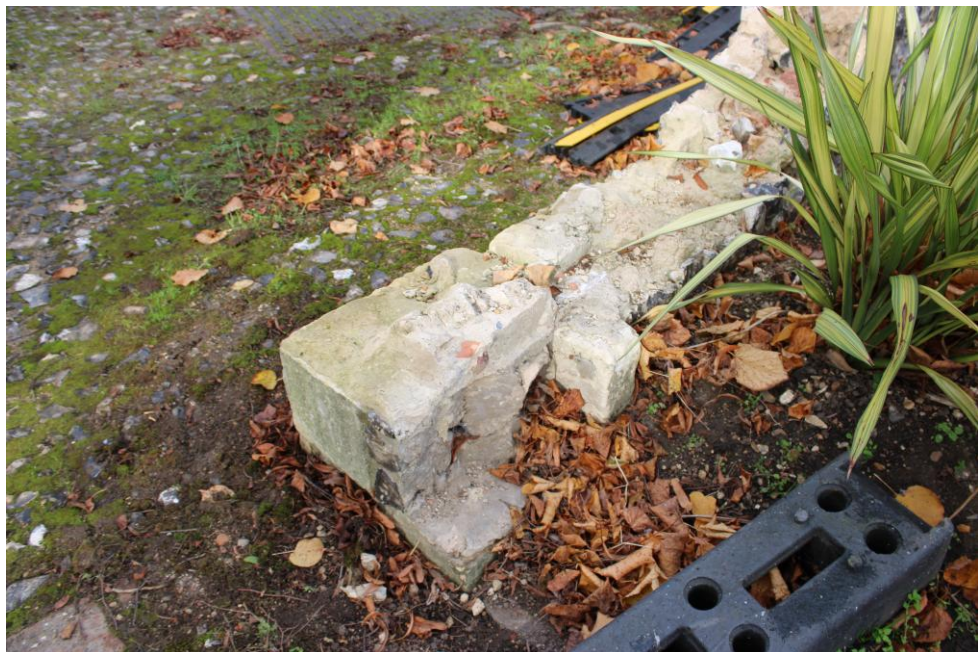
Fig. 3.3 Remaining pier and wall at lowest point
