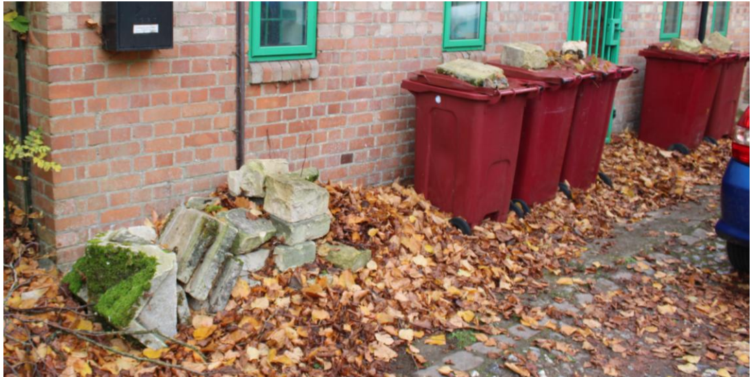
Fig. 3.2 Storage of materials from damaged wall
