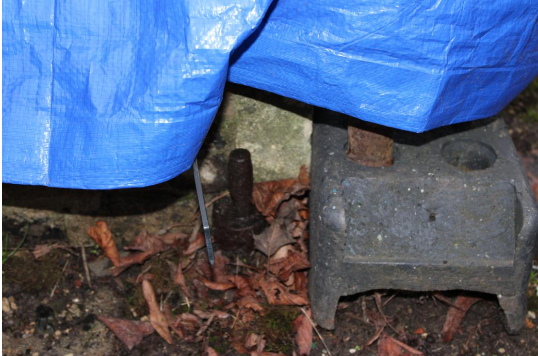
Fig. 3.8 North wall pier – lower gate pin
