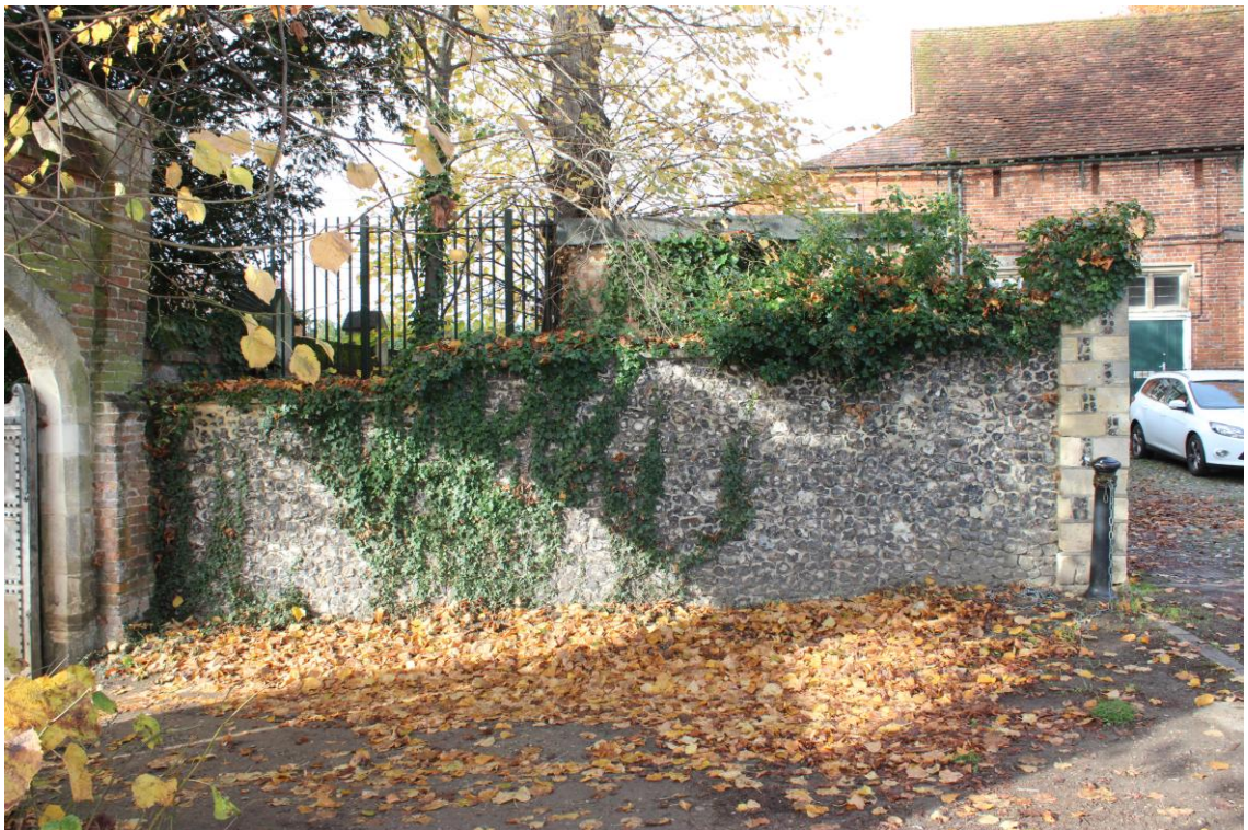
Fig. 2.3 Courtyard Wall, East elevation, south section (un-damaged)
