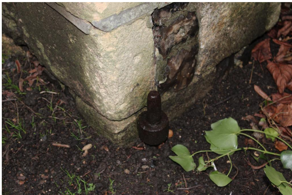
Fig. 3.8 South wall pier – lower gate pin
