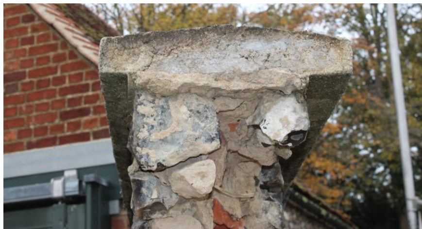
Fig. 3.5 Stone coping cross section
