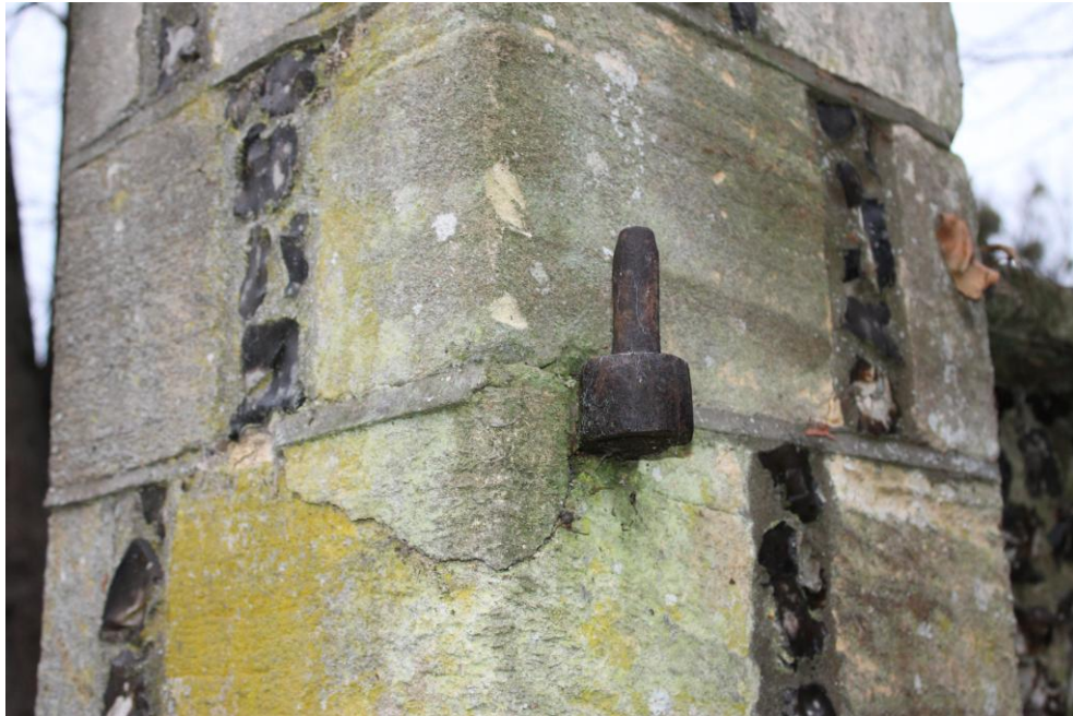
Fig. 3.7 South wall pier – upper gate pin
