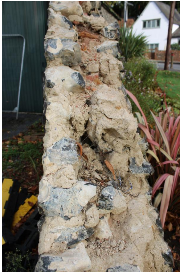
Fig. 3.4 Close up of wall construction through width
